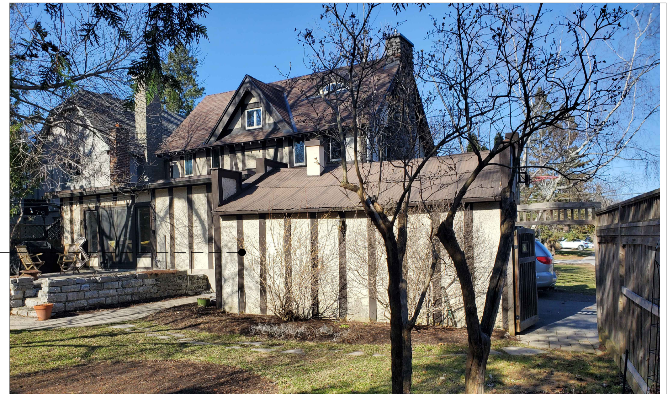
VIEW FROM REAR YARD
