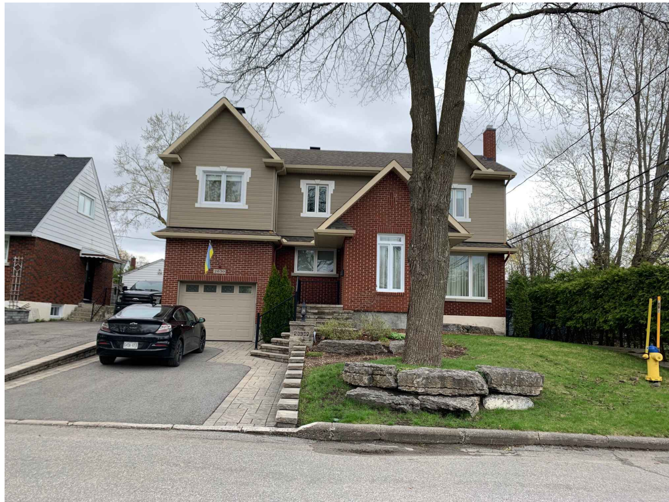
IMAGE 6A - EXAMPLE OF NON-CONFORMING PROPERTY: 2030 VINCENT STREET
