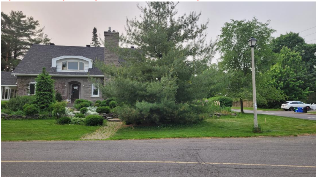
Figure 1-3: Existing dwelling at 1469 Portal Street, looking south
