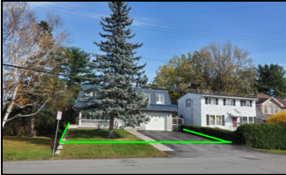
Image showing the front facade of 429 Ancaster Ave. from the street looking east.
