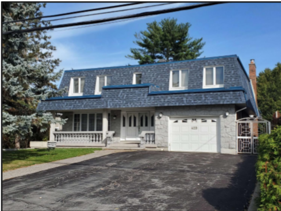
Image showing the front facade of 429 Ancaster Ave. from the driveway looking northeast.
