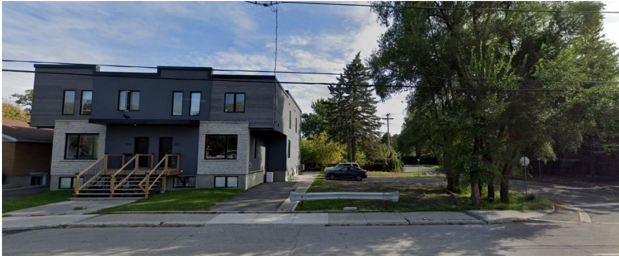
Figure 2 – Street view of the vacant lot at 1558 Baseline Road
