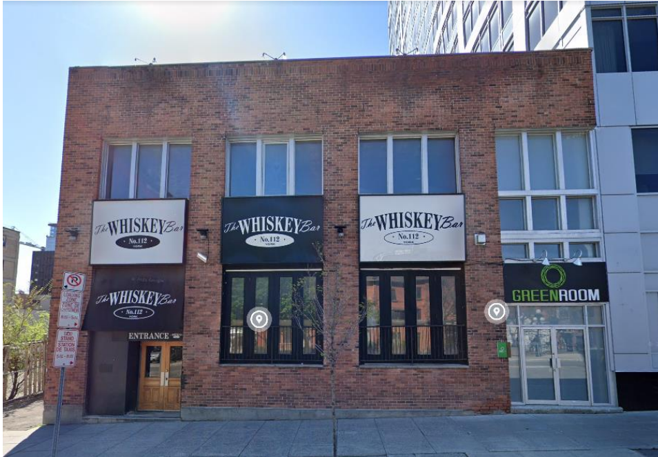
110 York Street, front façade
