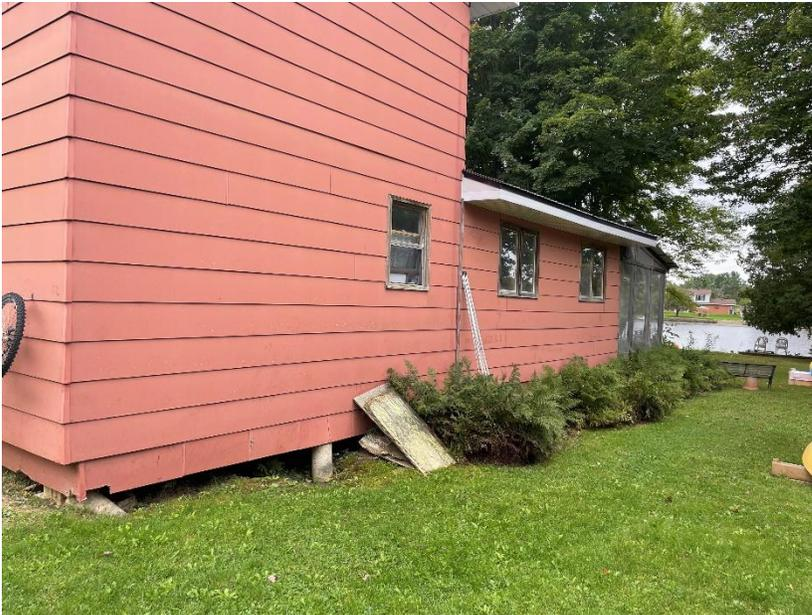
*2490 B River Road\_ Existing deteriorating sono-tubes foundations, September 2022*
