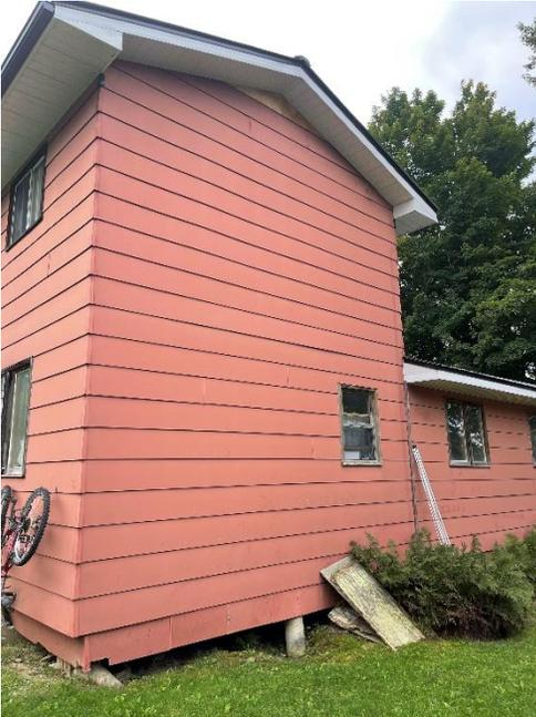
*2490 B River Road\_ Existing deteriorating foundations (Sono-tubes), September 2022*
