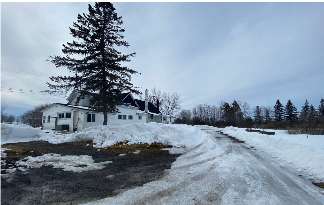
Figure 4: Existing house on subject property and access
