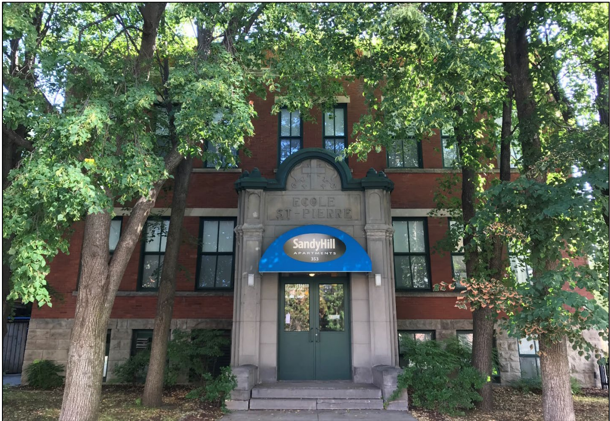
Top photos: Front elevation of 353 Friel Street (City of Ottawa, 2022); bottom photo: front elevation of 353 Friel Street (City of Ottawa 2019).
