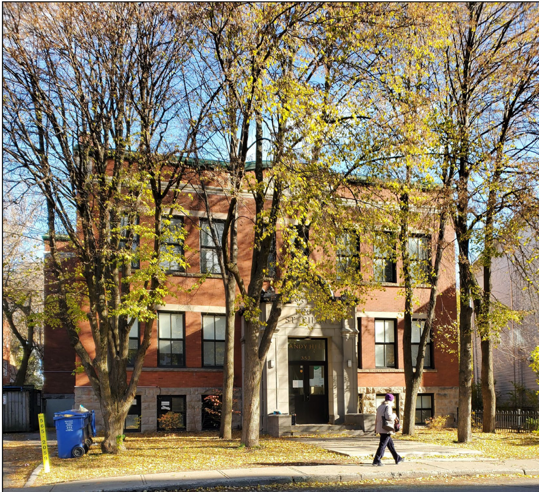
Figure 1: 353 Friel Street, front elevation; 1930 rear addition visible (City of Ottawa, 2022)
