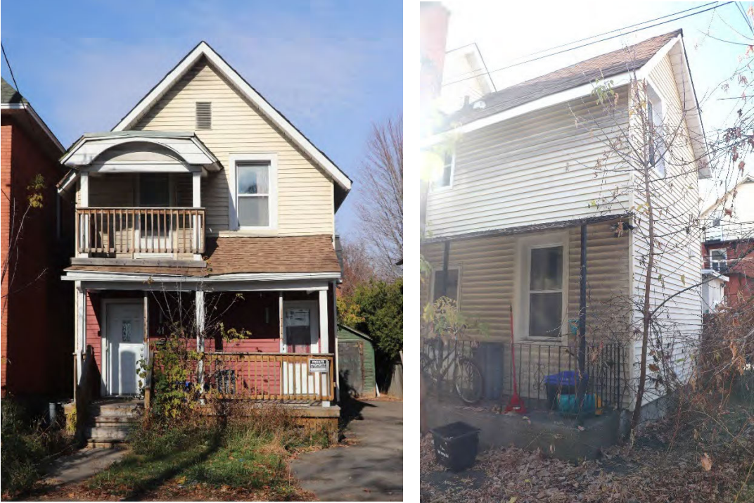
Figure 6: Façade (south) and rear one-and-a-half story wing (east and north elevations). (Heritage Studio, November 2022)
