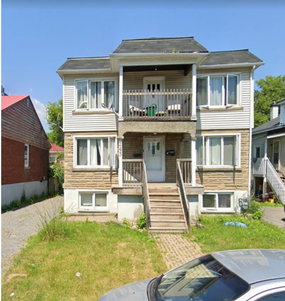
243 Ferland Street – multi unit building
