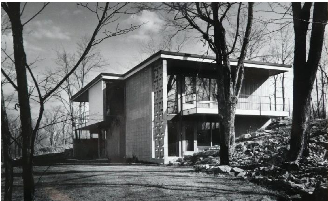
Figure 10: Cantilevered elements on the south façade (Library and Archives Canada 2022; ZMS Fonds; 3266-02)
