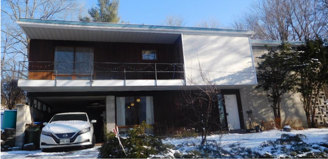
Figure 8: West Façade (City of Ottawa 2022)
