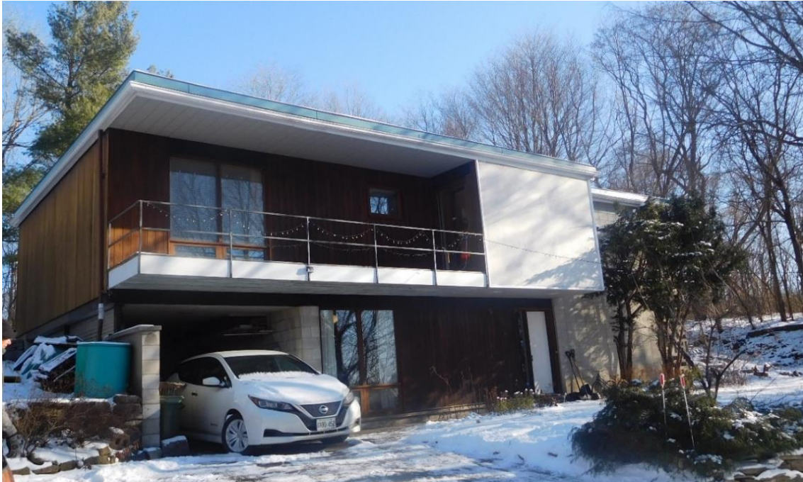
Figure 9: Cantilevered Elements on the West Façade (City of Ottawa 2022)
