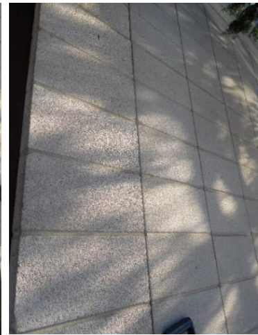
Figure 28: The concrete breeze blocks complement the surrounding rocky landscape (City of Ottawa 2022)
