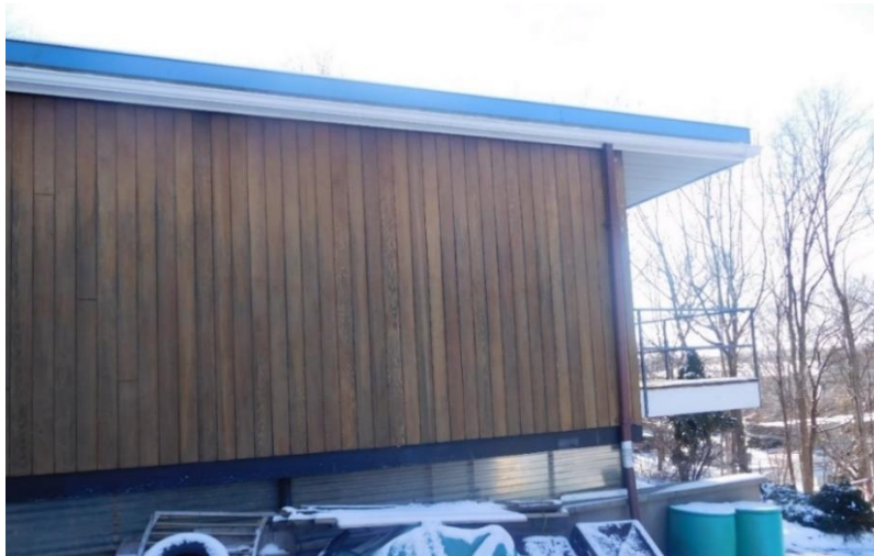
Figure 5: North Façade (City of Ottawa 2022)
