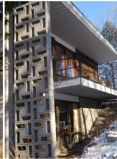
Figure 17: South Façade displaying the brise-soleil and integration of the property into the natural landscape (City of Ottawa 2022)
