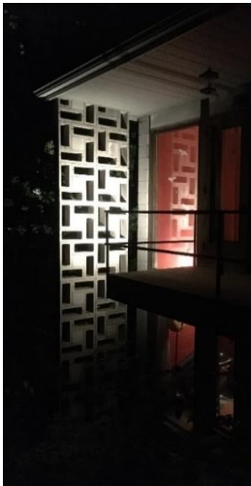
Figure 11: The brise-soleil as seen during the nighttime (Image provided by the current owner P. van der Roest & B. de Bruijn)
