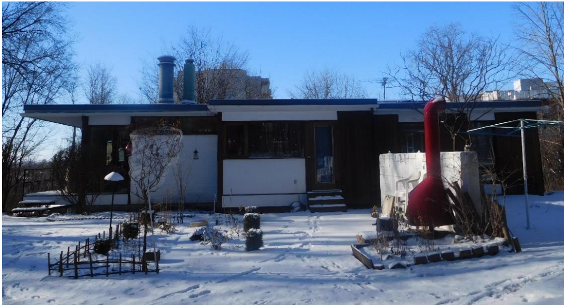
Figure 7: East Façade (City of Ottawa 2022)
