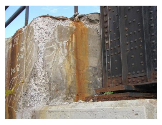
Abutments and piers exhibit severe to very severe delamination and disintegration of concrete encasement
