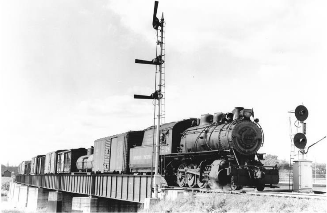
Figure 4: Bridge in service (Paterson & George, 1956)
