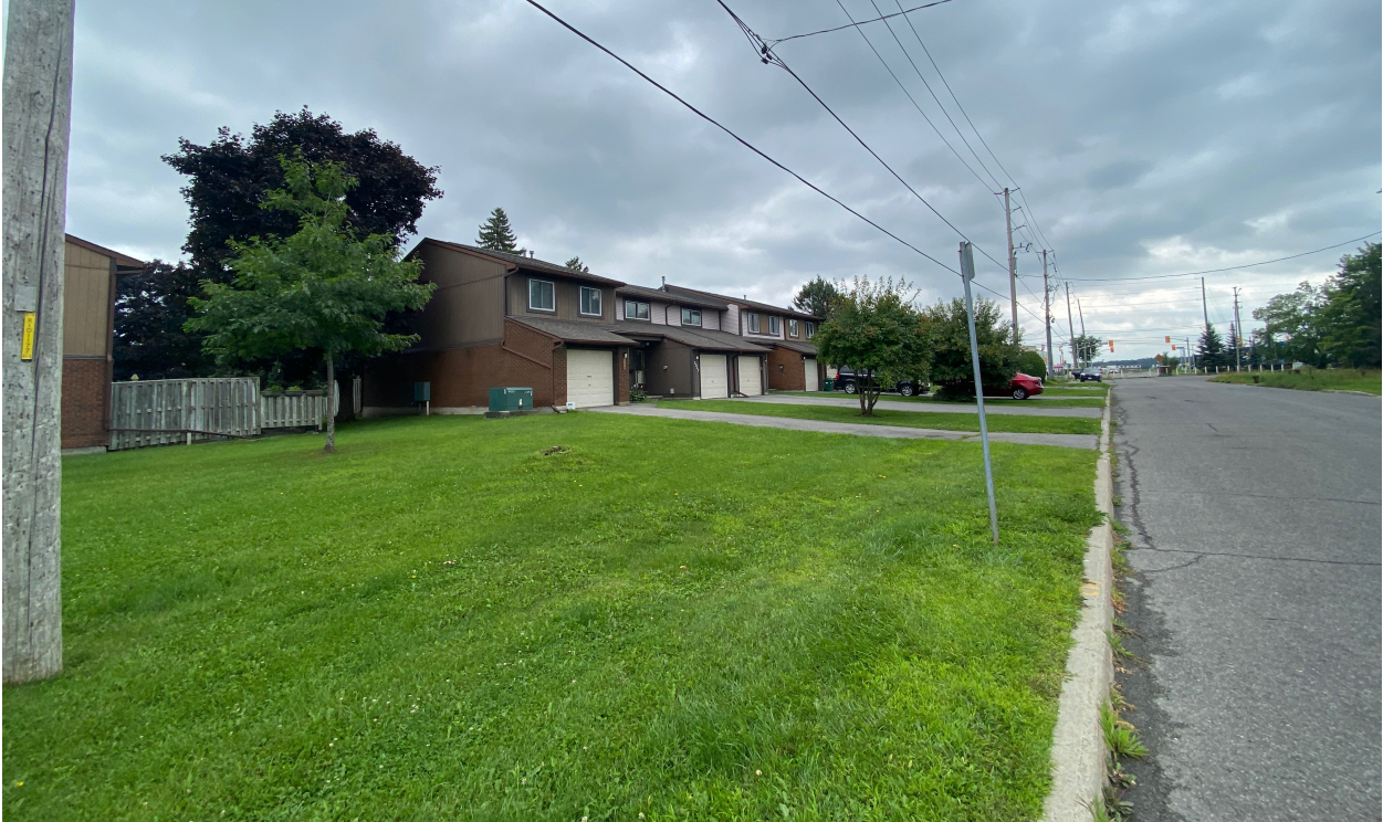
Figure 10: Townhouse development at Boyer Road and Mary Jane Crescent, south of the subject site
