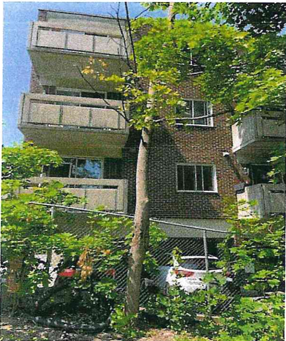
Tree #5, Norway Maple with rotten area on main trunk, to be removed.
