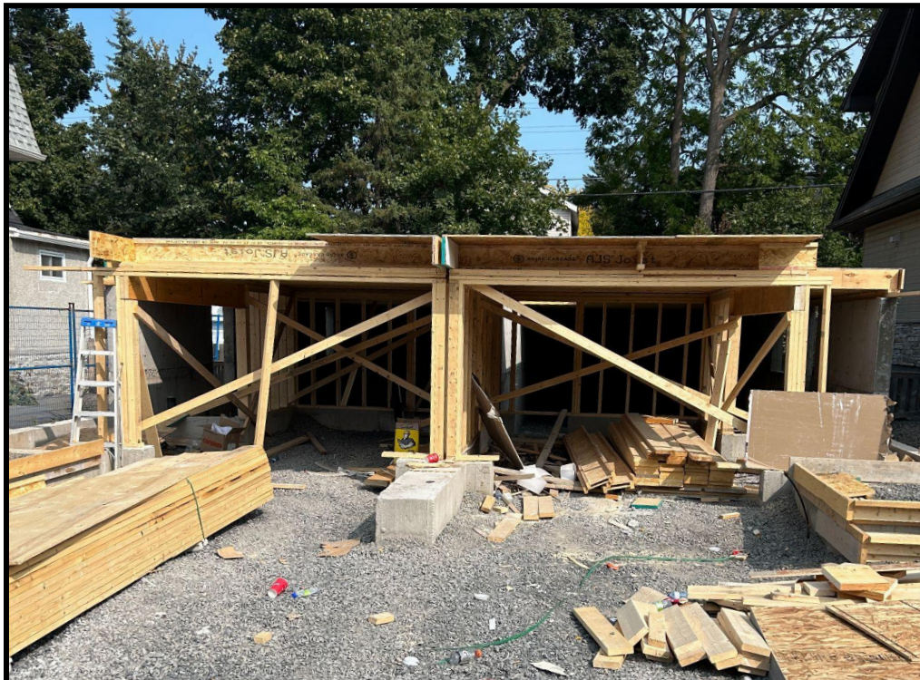
September 2023 imagery showing the semis under construction
