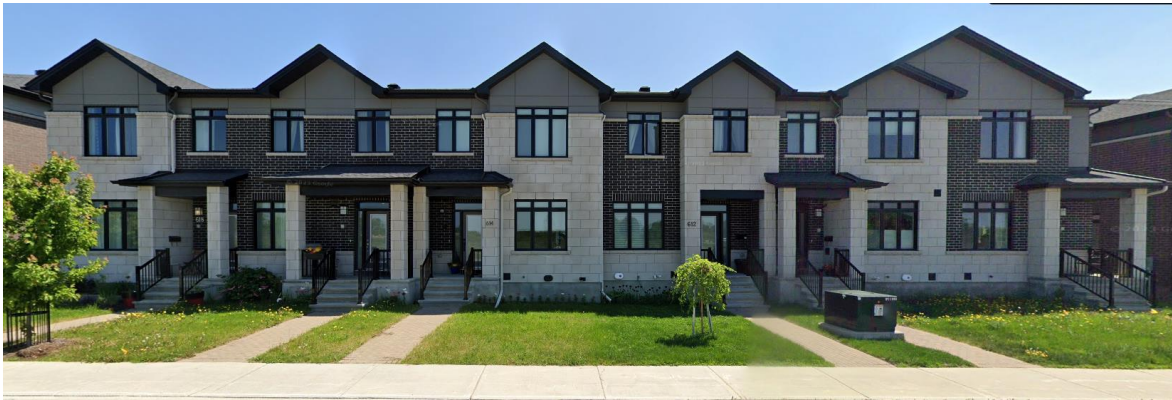
Figure 18: Façade of 608-618 Mikinak Road, diagonal to the subject site.
