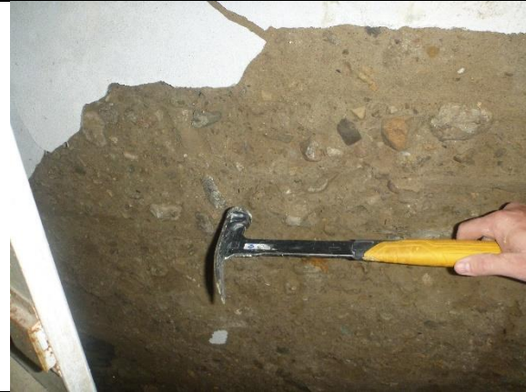
Photo 8: Soft concrete in the interior of the foundation wall [JCAL 2021]
