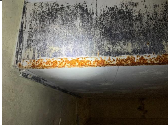
Photo 22: Typical extent of mold throughout basement [JCAL 2021]
