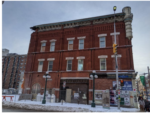
Figure A2 – North Exterior Wall
