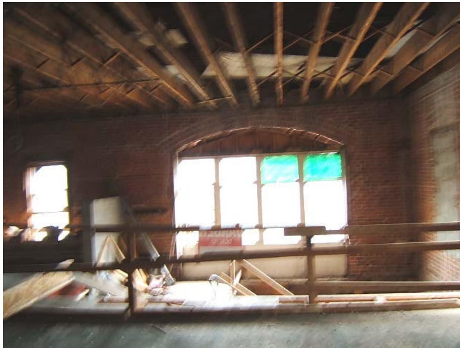
Figure 9: Previously Existing Condition Outlining Roof Diaphragm
