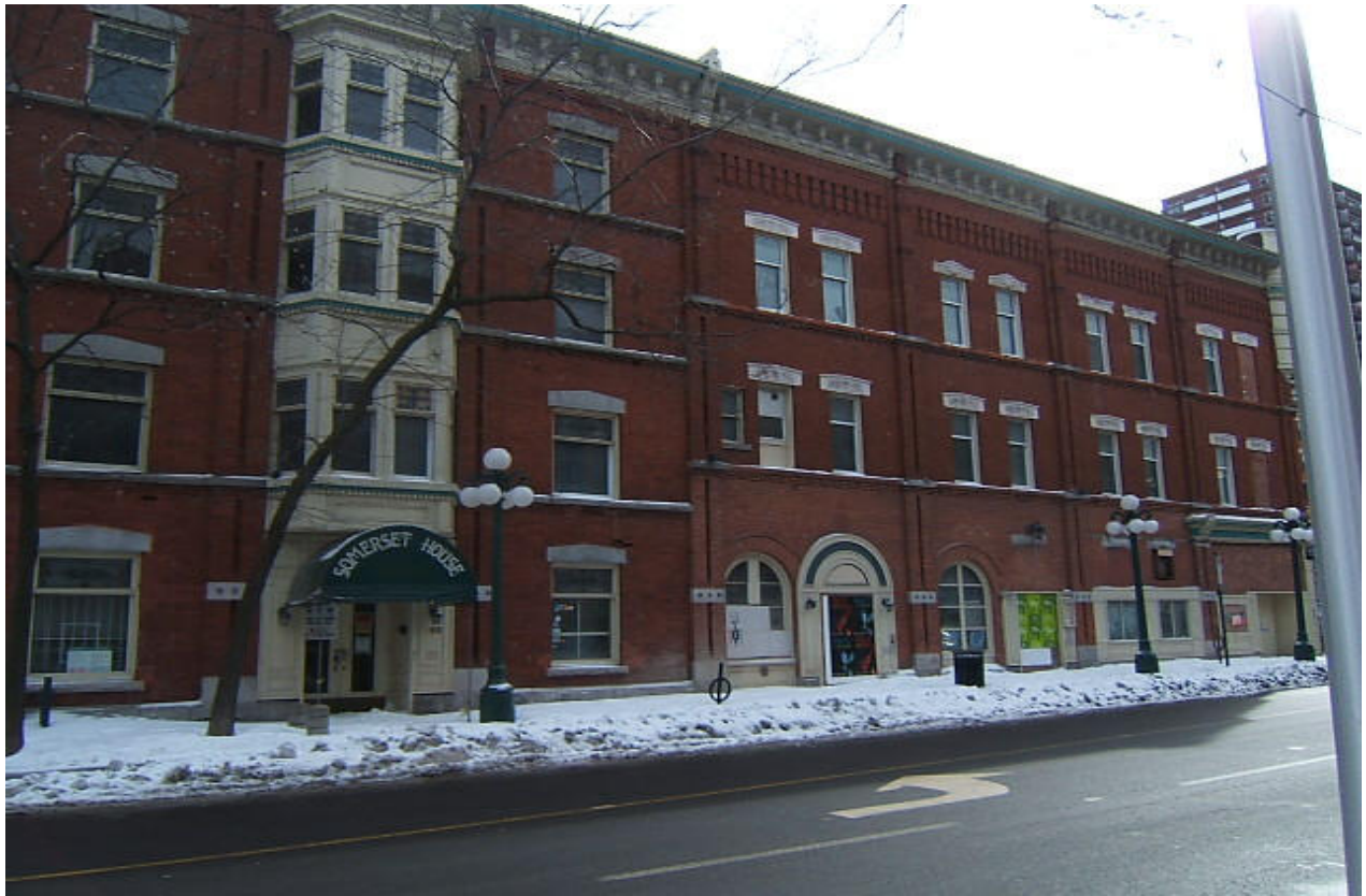
Figure 2: Previously Existing Condition Showing Eastern Addition
