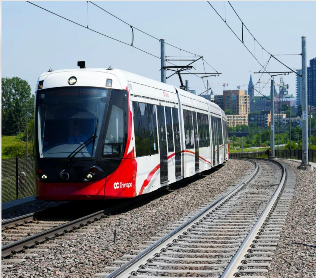
Figure 4 – Image Showing Typical Sections of Track, Catenary and LRV:
