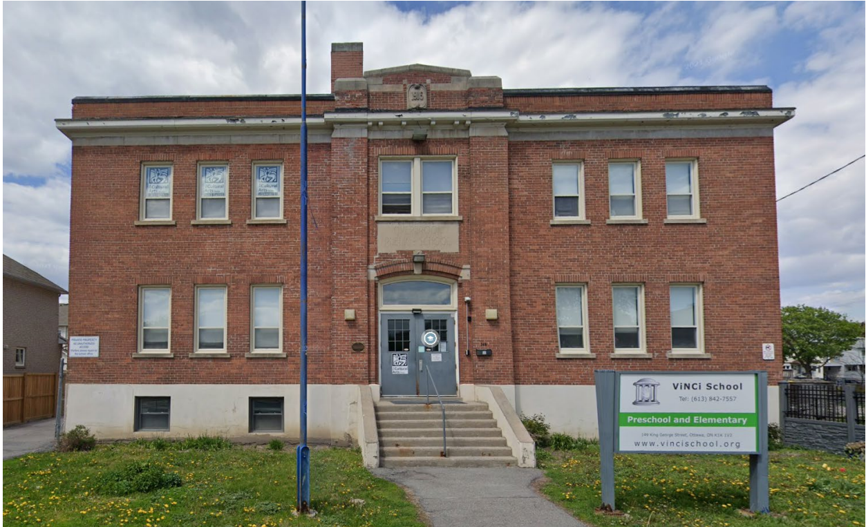
Front façade of 149 King George Street
