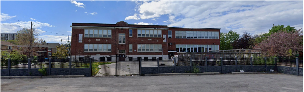
Side (east) façade of 149 King George Street
