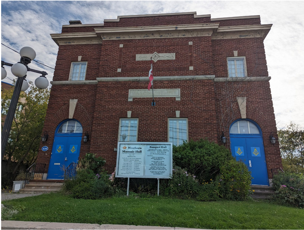
Front façade of 430 Churchill North, looking west (City of Ottawa, 2023)
