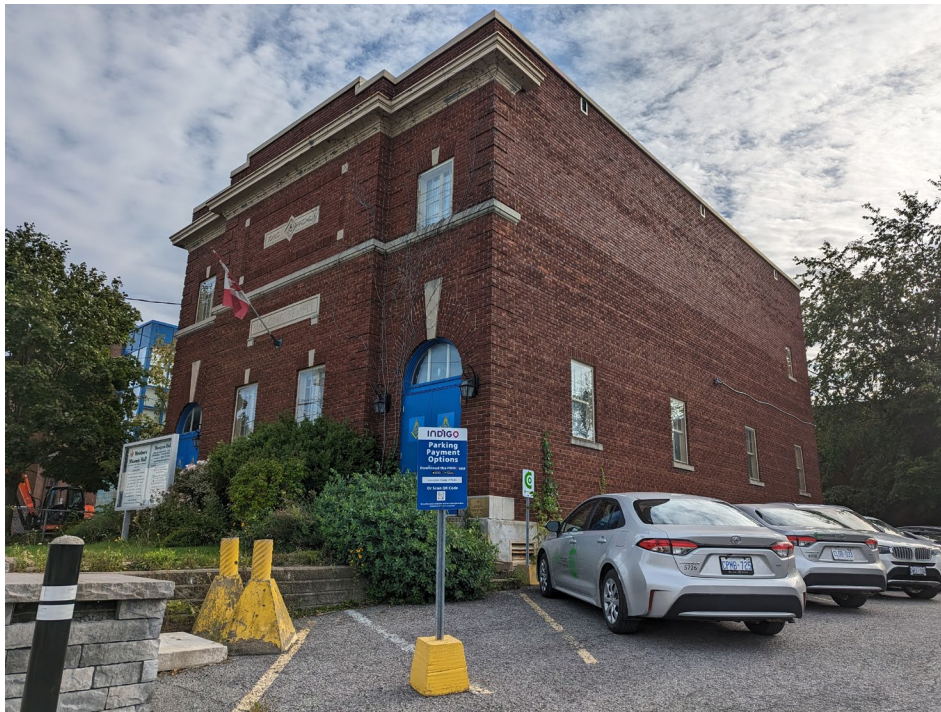
Front and North façade of 430 Churchill North (City of Ottawa, 2023)
