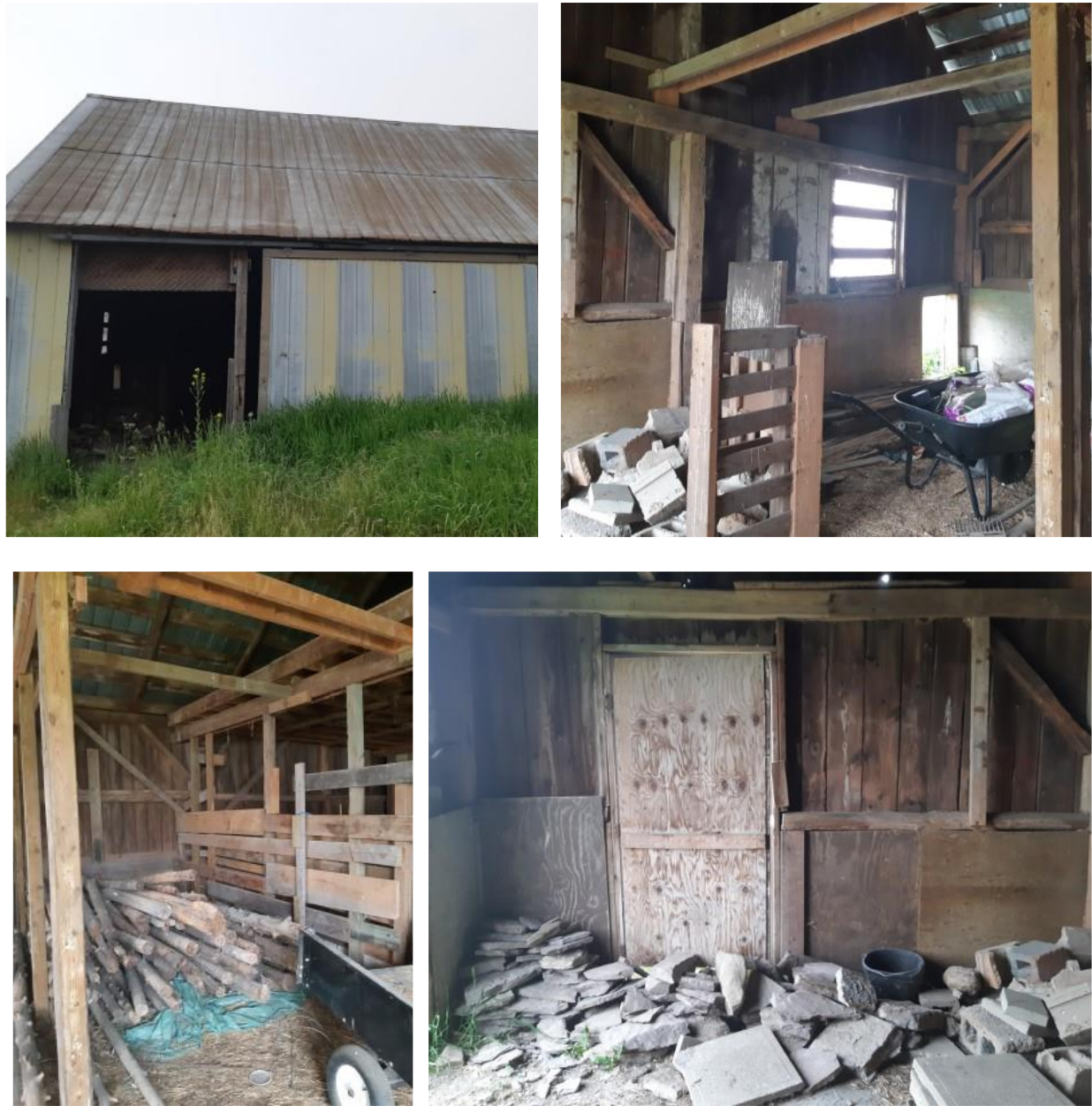
Figure 2: The exterior and interior of the vacant barn on the Subject Site (Novatech, June 2023).
