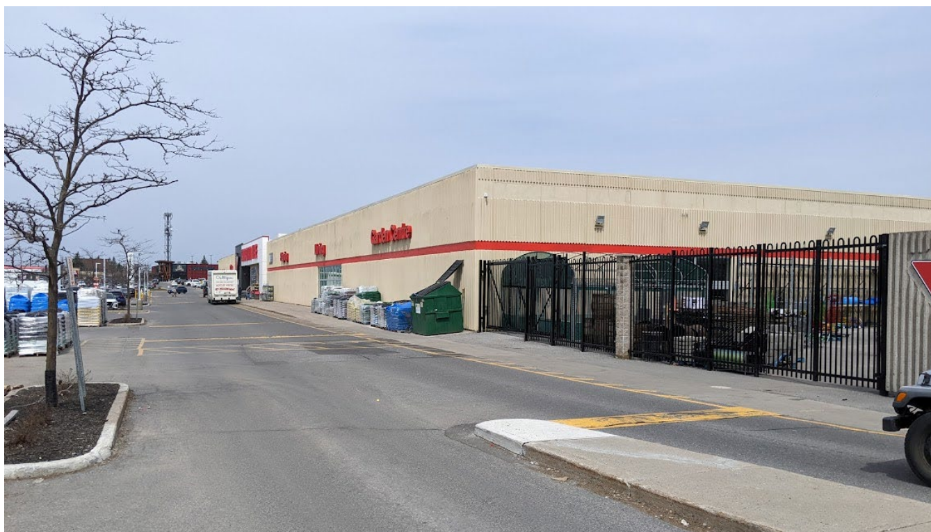
Photo 2: View of existing garden centre and frost house area, looking northeast towards the main building entrance (Parsons, April 2023).
