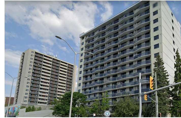
3. HIGHRISE MULTI-UNIT APARTMENTS ON CARLING
