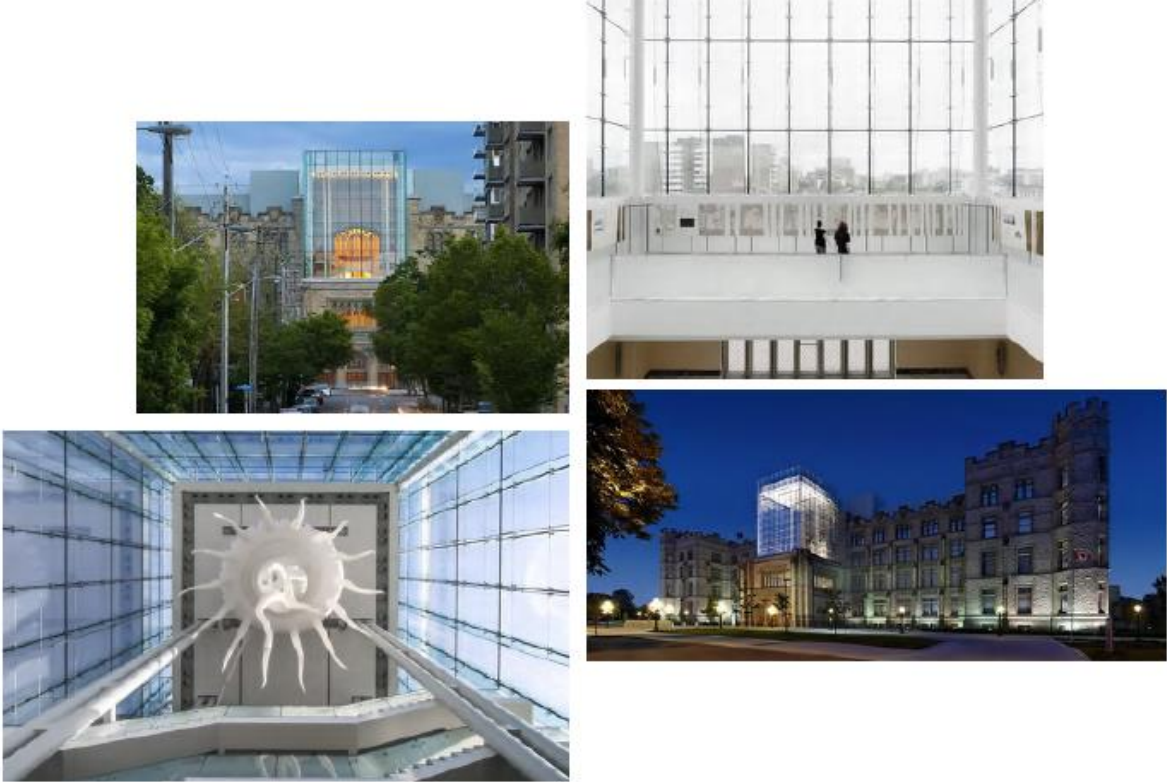
Figure 6: A contextual view looking south towards the main entrance of the Museum of Nature. The Museum set in a park provides a distinct precinct for the buildings surrounding the open space.
