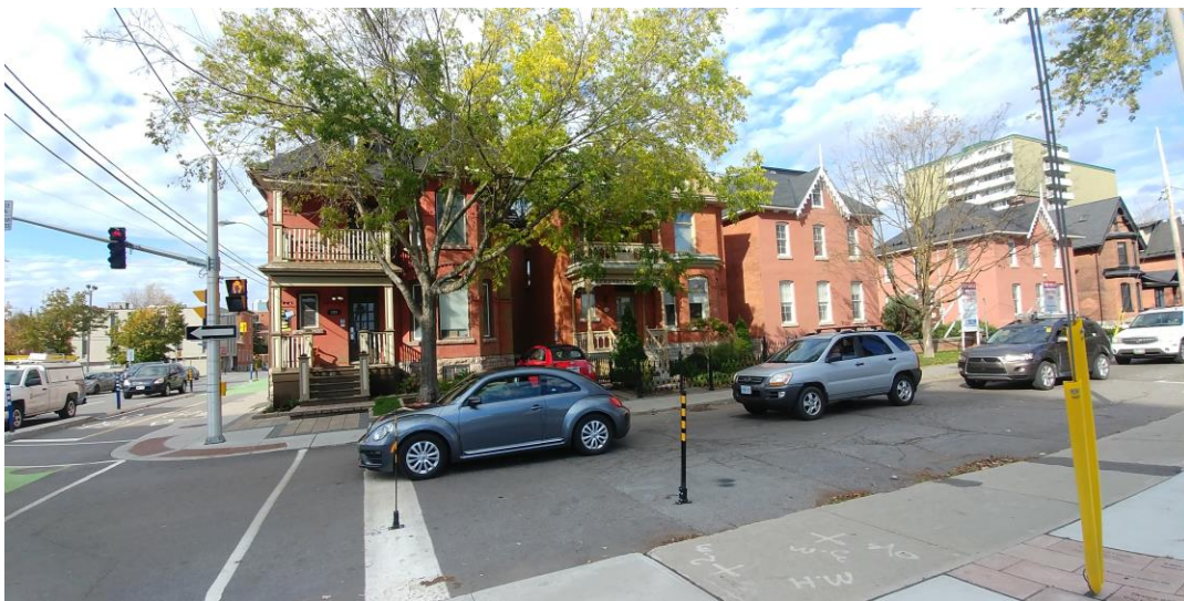
Figure 3: Context view looking north at the intersection of O’Connor. At O’Connor, the grouping of two identical buildings define that corner. The third building in this grouping 385 McLeod was altered. The 12-storey high-rise framing the block at O’Connor and Gladstone is very visible. The 8-storey unit directly behind the subject property is not intrusive from this view. Source: Google Maps
