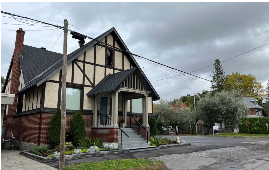
Front façade of 415 Kenwood Avenue
