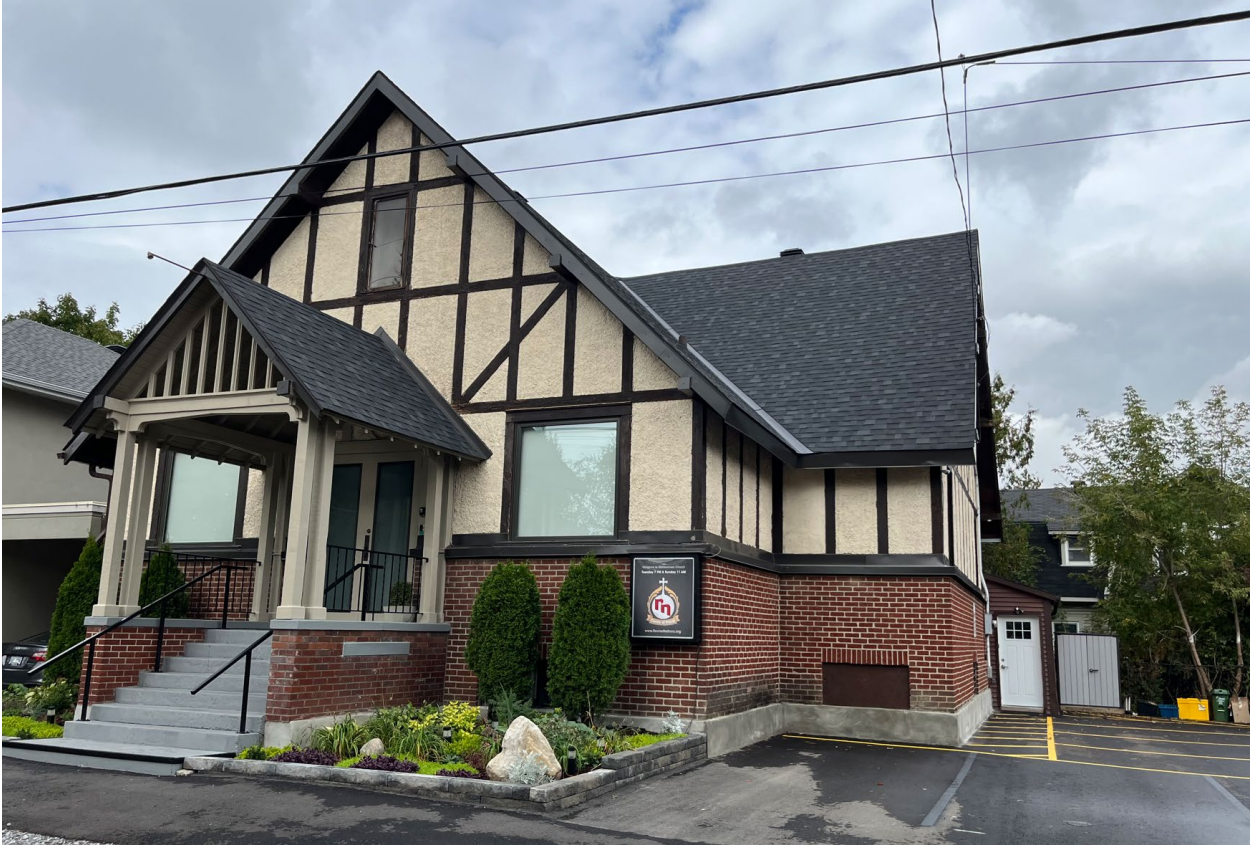
Front façade of 415 Kenwood Avenue
