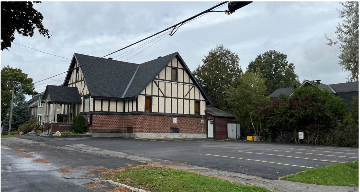
View of 415 Kenwood Avenue from Kenwood and Roosevelt Avenues
