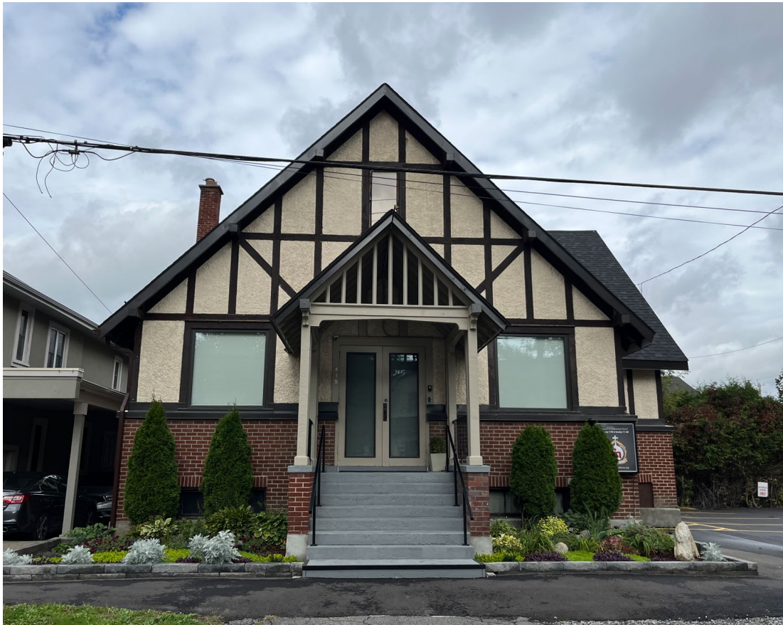
Front façade of 415 Kenwood Avenue
