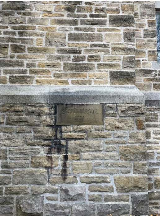
Southminster United Church 1931 Date Stone. Source: City of Ottawa
