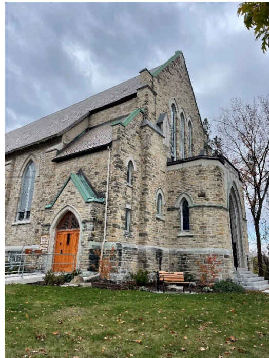
Southminster United Church, South Entrance Source: City of Ottawa
