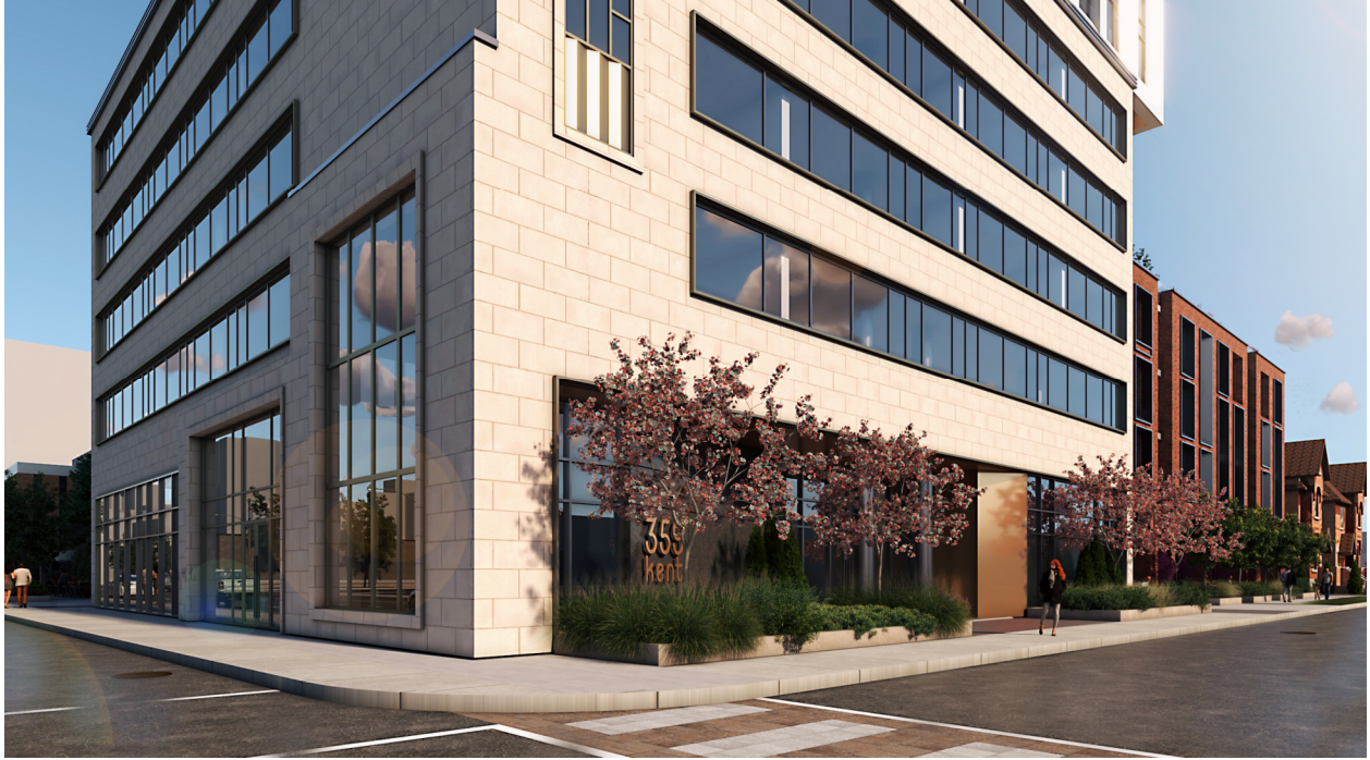
Figure 22: A rendering detailing the treatment of the renewed entrance at Kent and Gilmour Streets.
