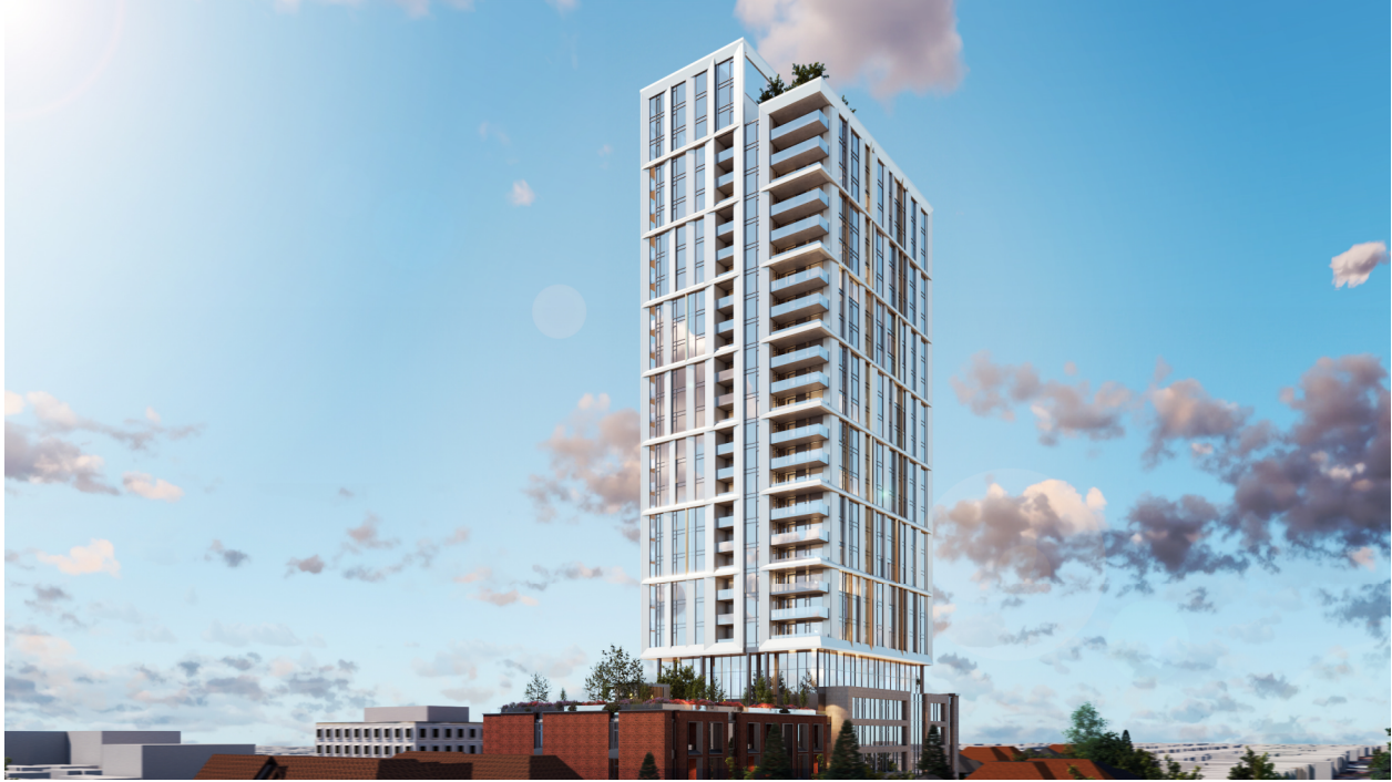
Figure 16: The Legion Building serves as a podium that steps down to 4 storeys along Gilmour and helps integrate into the neighbourhood. The 20-storey tower setback from the street is positioned to allow the reconstructed Legion façade to stand proud. The tower designed as the beacon acting as a guide to the downtown core will also be visible as a new iconic piece in the Ottawa skyline from the Queensway. Source: Hobin Architecture July 2023.
