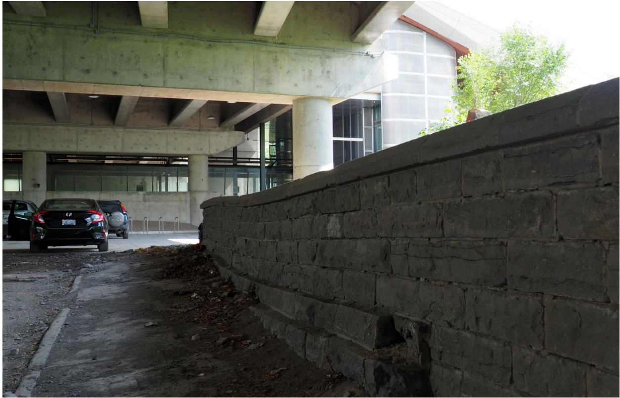
Figure 8: Looking south from Old Booth Street towards the new Pimisi LRT station, June 2019. Source: Contentworks.
