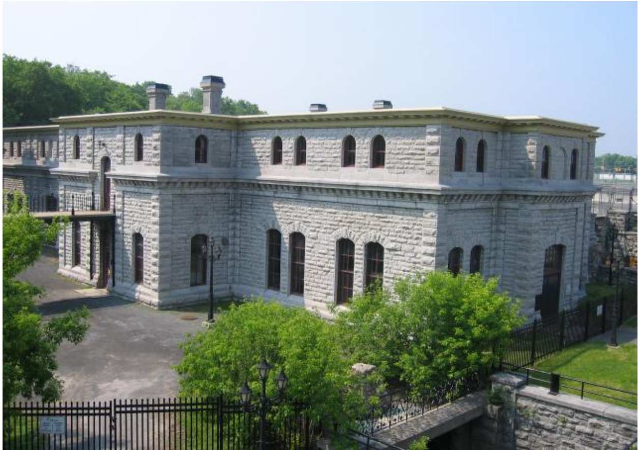
Figure 5: Fleet Street Pumping Station, originally designed as a one-storey limestone masonry building by Thomas C. Keefer. Pumping capacity was increased in 1888 when new machinery was installed in an addition designed by architect E.L. Horwood, who also replaced the original mansard roof with a second storey. Source: James R. Skinner/Wikipedia, 2006, https://en.wikipedia.org/wiki/Fleet_Street_Pumping_Station#/media/File:FleetStreetPumpingStation.png .
