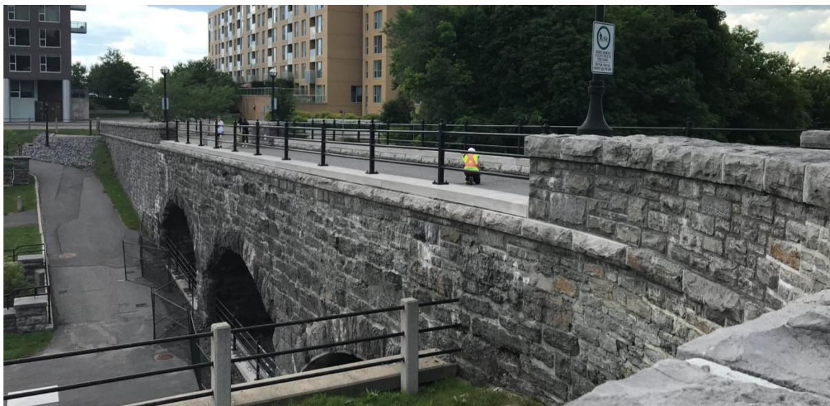
Figure 11: Pooley's Bridge, south arches, June 2019. Source: Contentworks.
