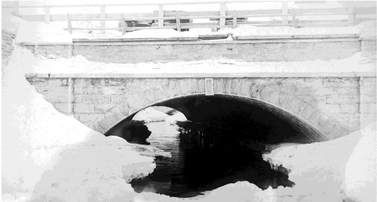
Figure 18: Looking west towards the east spandrel of the Lett Street Bridge, 1903. The parapet is much shorter than it appears in the 1911 photograph and may have been under construction to be raised when this photo was taken. Source: City of Ottawa Archives, Ottawa Water Works MG305, Accession 40D91.
