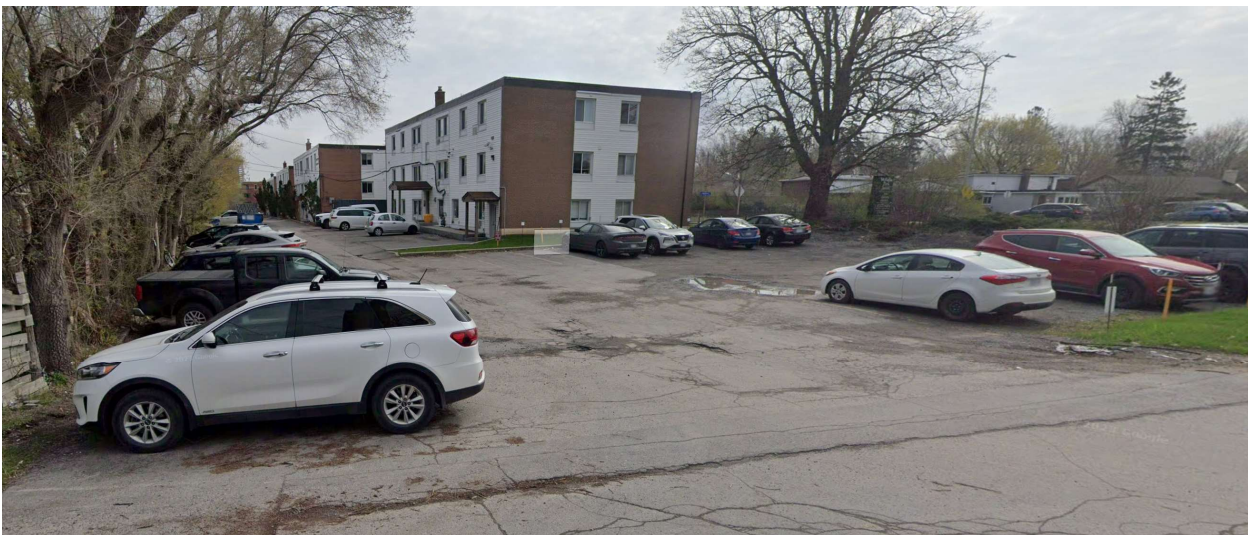
Exhibit D: Photographs of the Subject Property from Bromley Road (source: Google)
