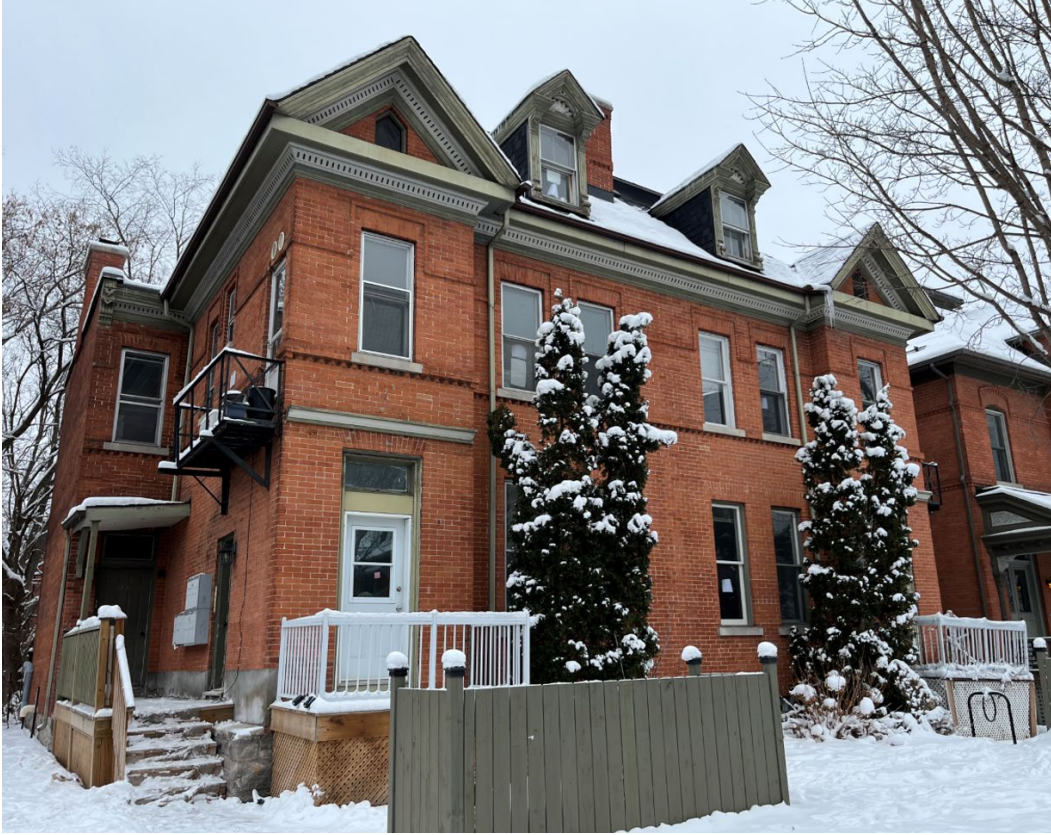
Front façade of 29 Russell Avenue
