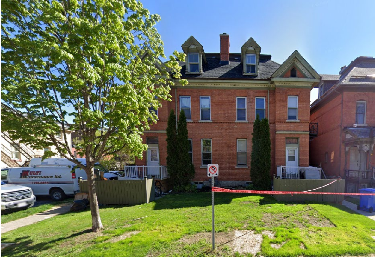
Front façade of 29 Russell Avenue
