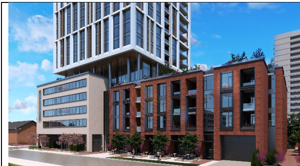
Figure 5: The 6 storey podia steps down to 4 storeys along Gilmour Street facade
