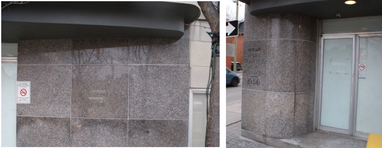
Figures 16 & 17: (6 -left) View of the introduced polished granite panels to the right of the Gilmour Street entrance. (7-right) View of the original polished granite panels. Source: Commonwealth 2023
