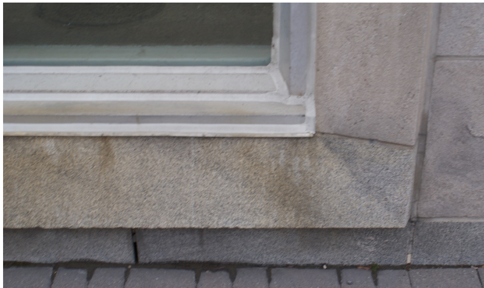
Figure 25: Detail of the granite plinth course and granite windowsill surround at the base of the three-storey Kent Street window. The colour of the granite sill is very close to the limestone cladding and window surrounds. Source: Commonwealth 2022.
