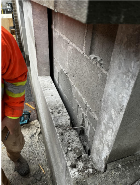
Figure 12: View of a test removal panel from a building at 100 Argyle constructed circa 1955 using a similar limestone cladding material as 359 Kent. The limestone cladding units are secured to the concrete block back-up wall with a single metal anchor centred on the width of the panel. Source: Heritage Grade Test Removal Report, 100 Argyle.
