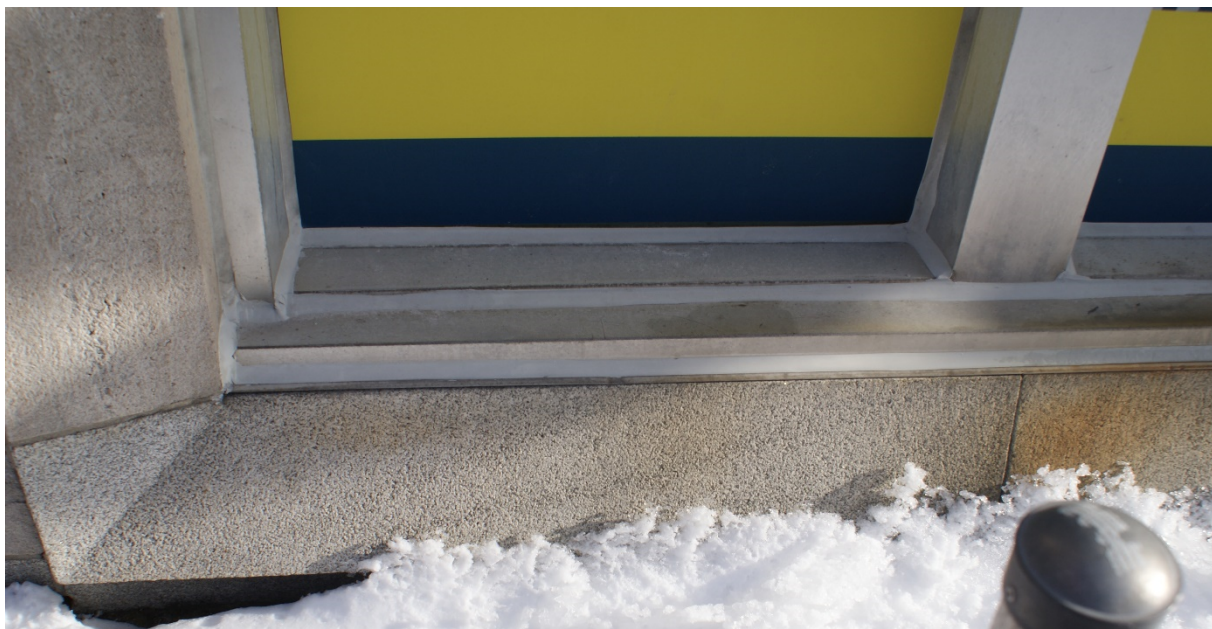
Figure 23: Detail view of the base of the Kent Street window. The horizontal units at the base of the window are formed of the same material as the granite plinth course. The vertical stone to the left is a limestone unit. Note the close match in colour and surface texture. Source: Commonwealth 2023
