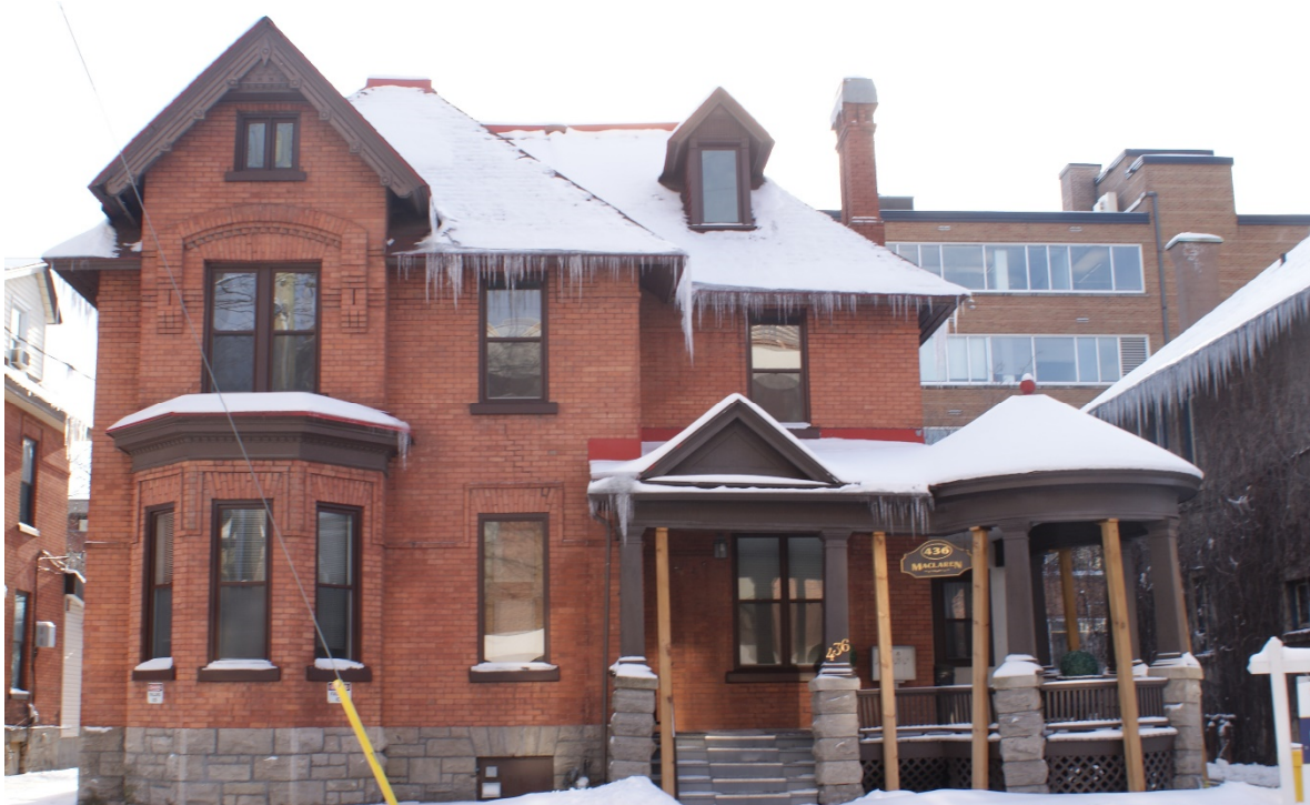
Figure 35: View of 436 MaClaren Street. The masonry piers supporting the porch have settled due to inadequate foundation depth. A detailed assessment of the condition of the porch is required. Guidelines from the CHCDP provide guidance for the conservation approach to the materials and assemblies. Source: Commonwealth 2023.
