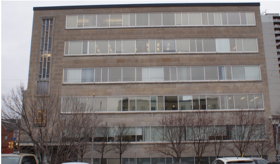
Figure 30: View of the windows on the Gilmour Street façade. All of the original windows have been replaced with the exception of the three-storey window above the Gilmour Street entrance. Source: Commonwealth 2022.
