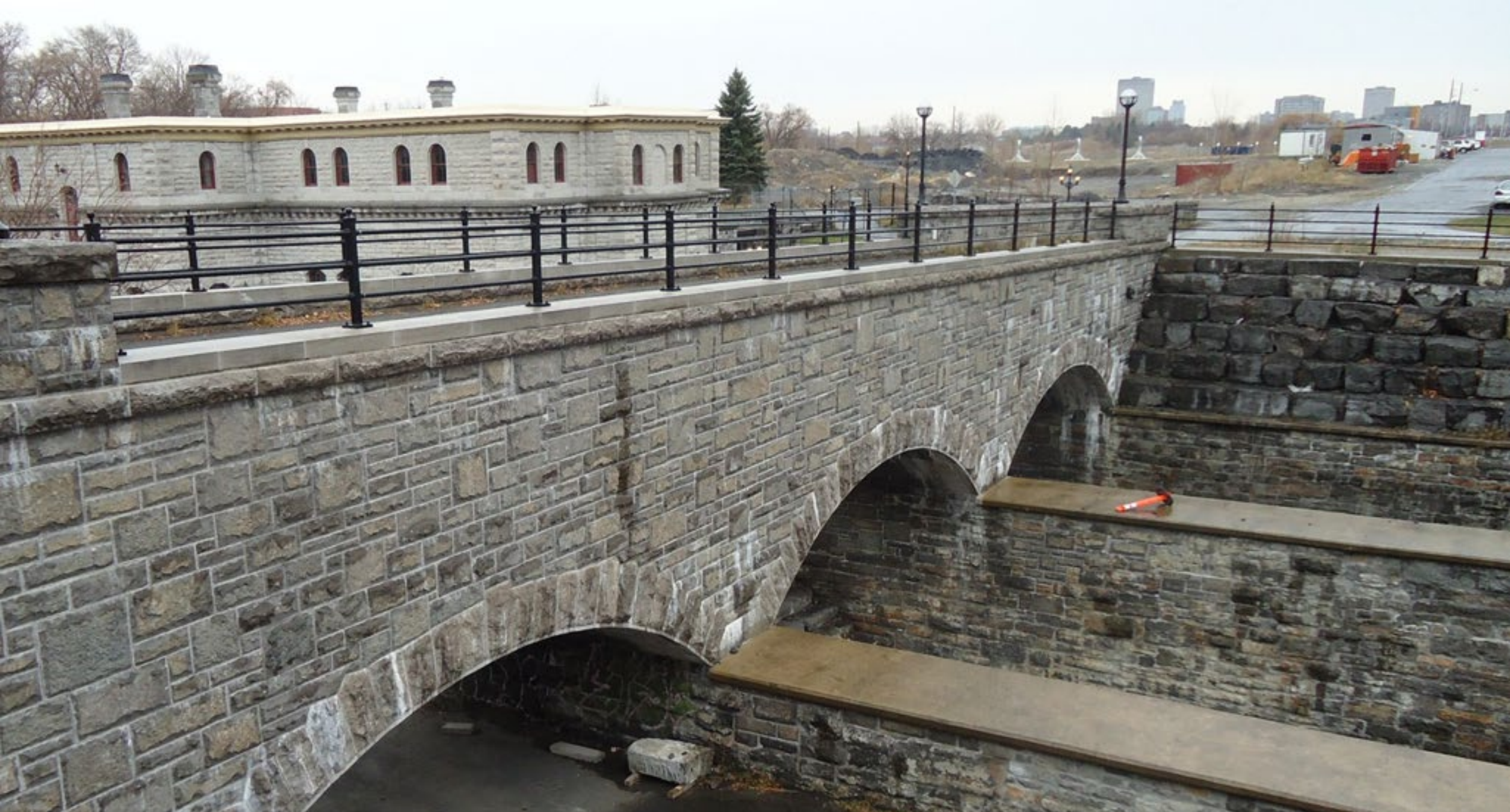
Pooley's Bridge and channeled tailrace. Jun 2016, City of Ottawa
