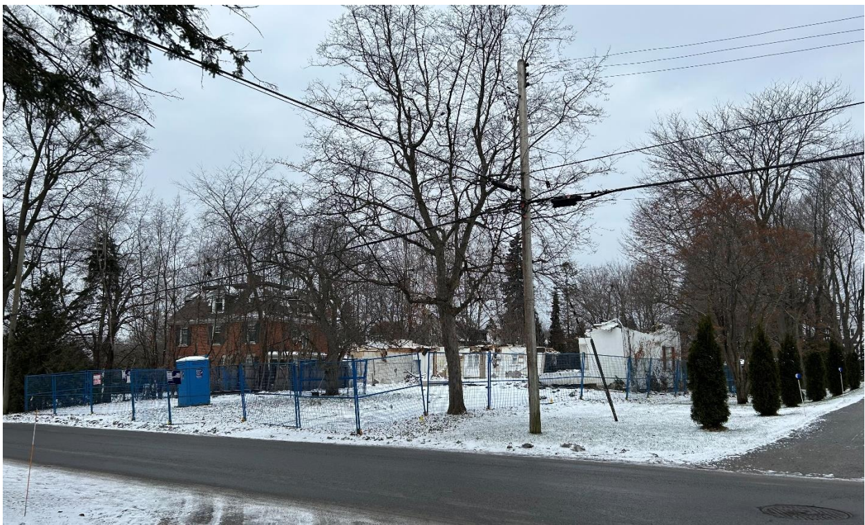
Current photo of the property, post demolition.
