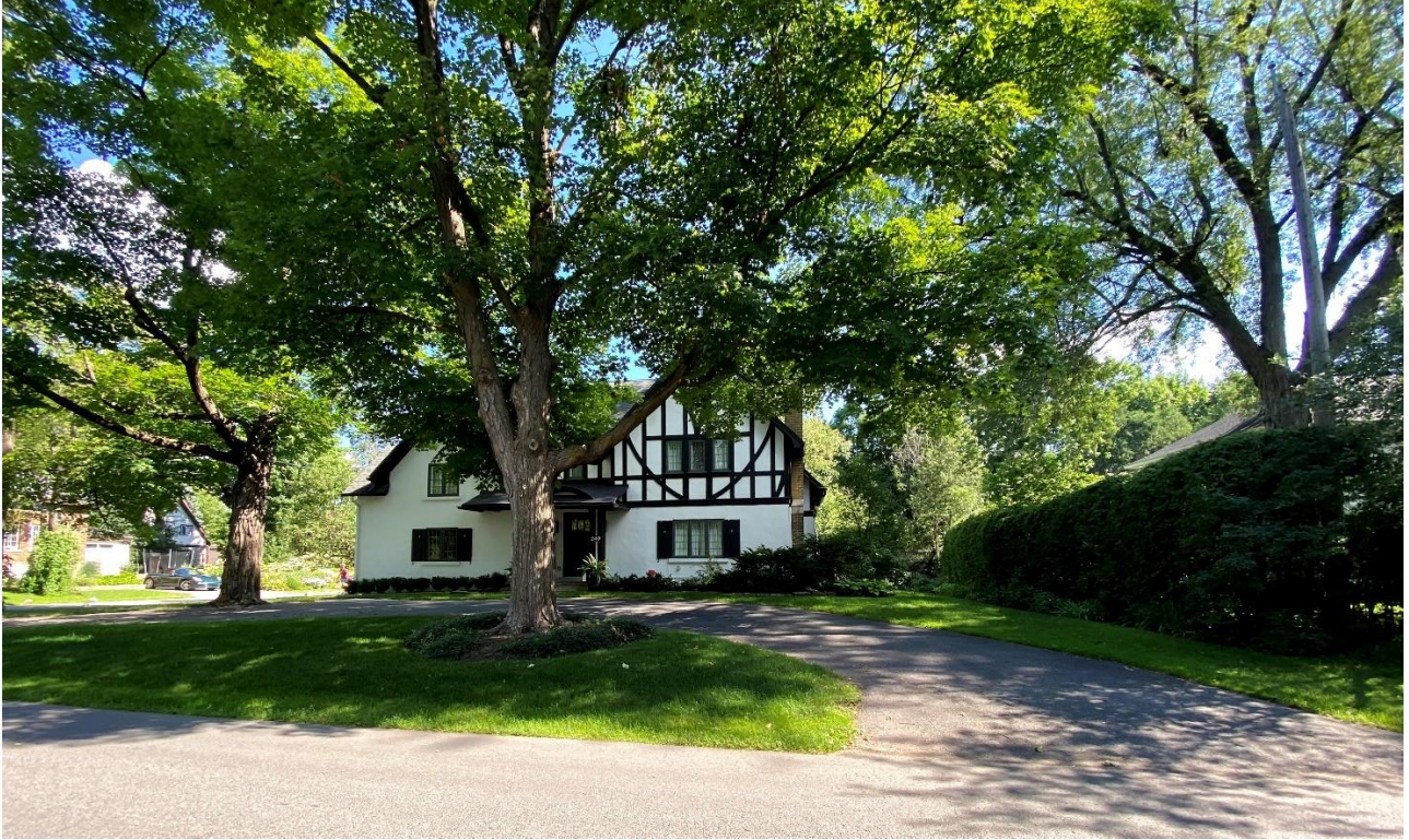
View of 240 Mariposa on the south side, across the street from the subject property.
