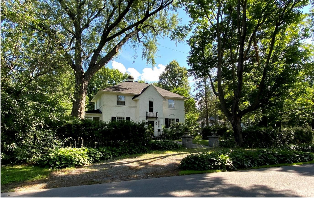
View of the 210 Mariposa on the south side, across the street from the subject property.
