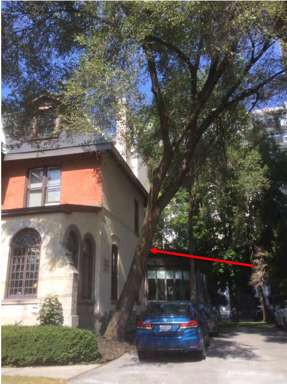
Photo 3: Tree E03 (remove) – Heavy leaner to east over existing driveway and conflicts with proposed accessible ramp.
