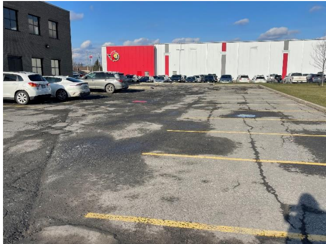
Photo of parking on east side of 839 Shefford Road
