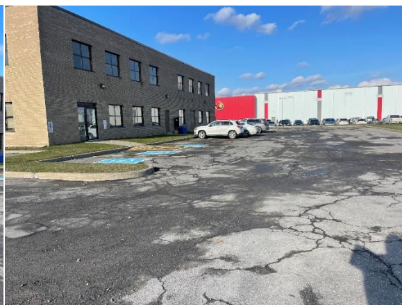
Photo of parking on east side
