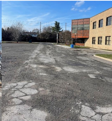
Photo of existing driveway
