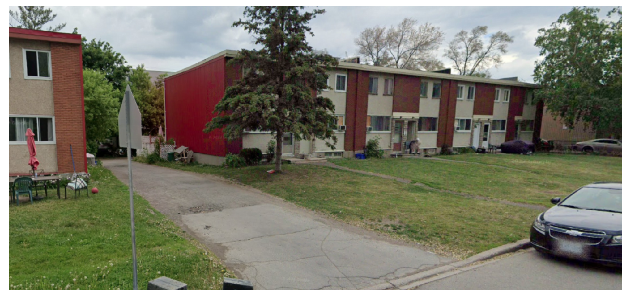
5) Exterior photo of neighbouring townhouse block 1293 Coldrey Avenue (right).
