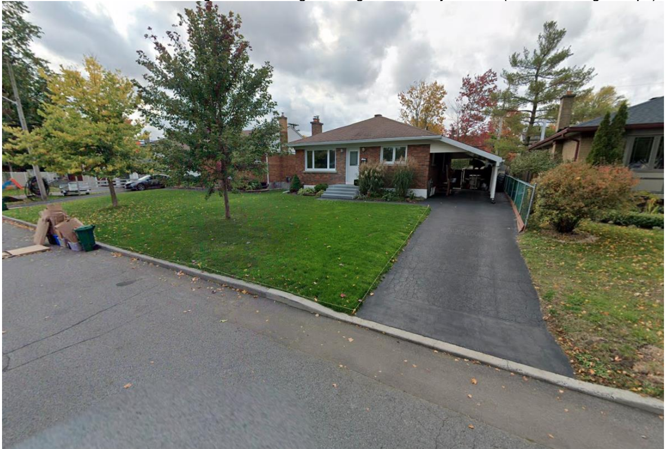
Figure 3: Existing Building on the Subject Site. (Source: Google Maps).
