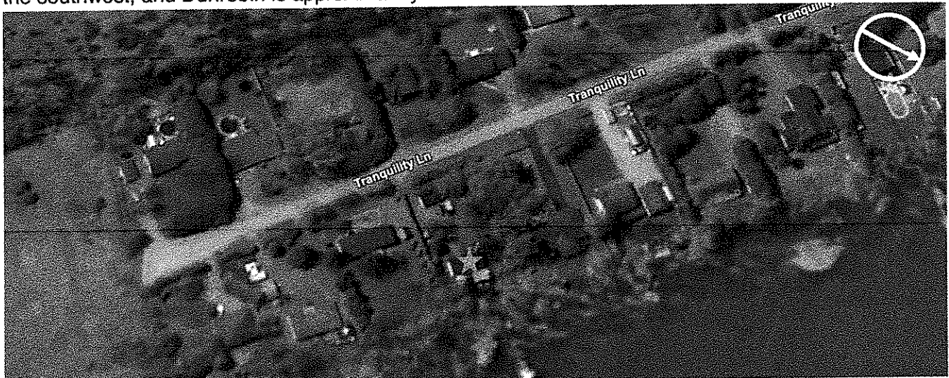
Figure 2. Aerial imagery of subject site and surrounding conditions (Google Earth, 2022)
