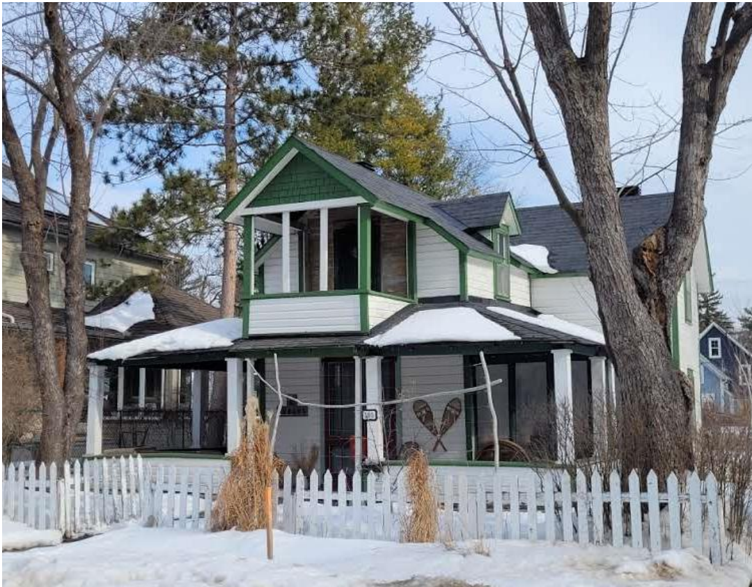
195 Bradford Street, west and south façade, Source: City of Ottawa, 2024
