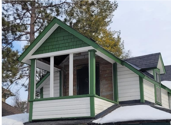
119 Bradford Street, second storey porch, Source: City of Ottawa, 2024
