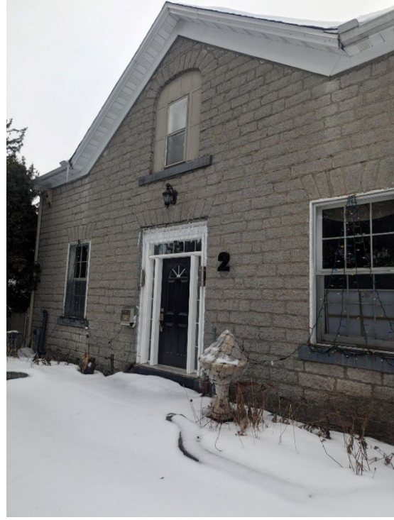
Large rectangular window openings with multipaned units in a 6 over 6 pattern at the east facade. Source: City of Ottawa
