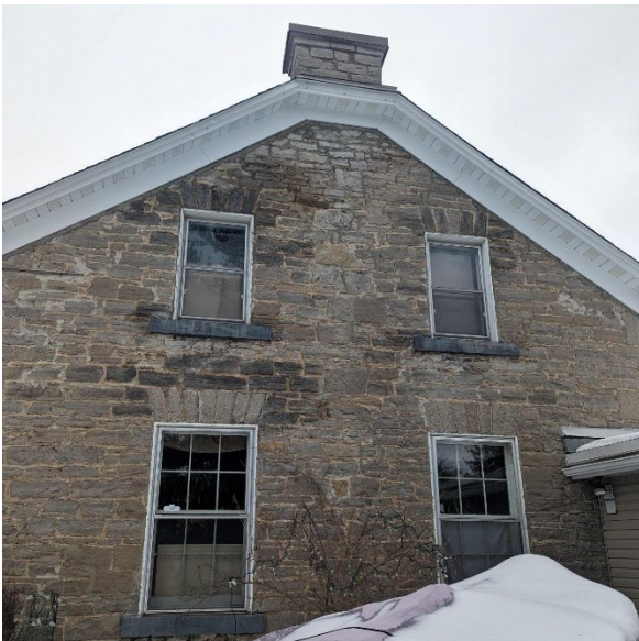
2 Peter Street stone sills and voussoirs. Source: City of Ottawa
