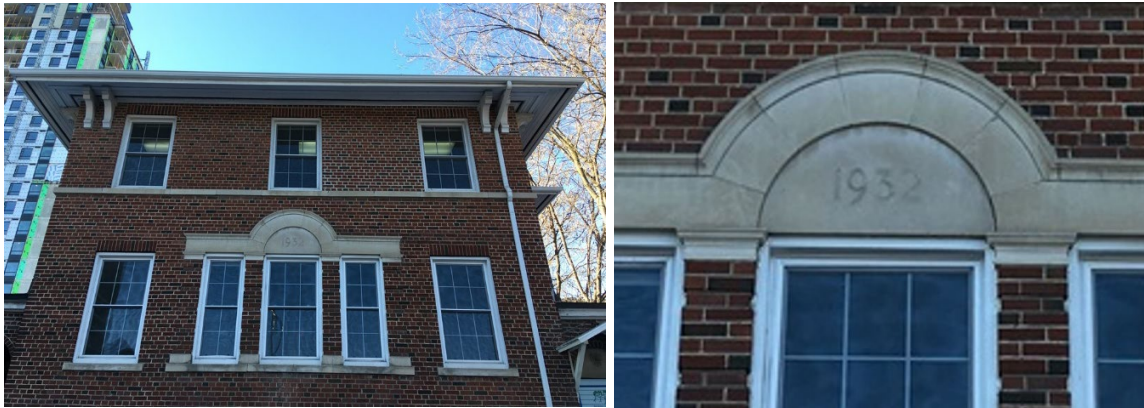
East elevation (left) and 1932 date stone (right).
