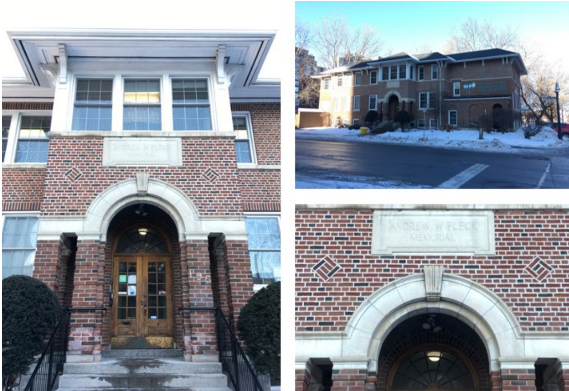
Views of the south façade, January 2023. Source: City of Ottawa.
