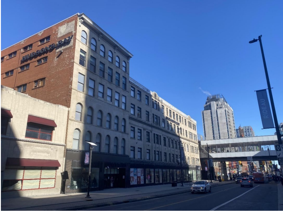
View looking north towards the pedestrian bridge connecting to the Rideau Centre. City of Ottawa, 2024.
