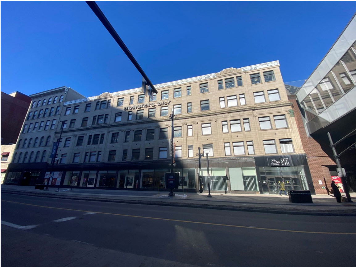
Front façade, City of Ottawa , 2024.
