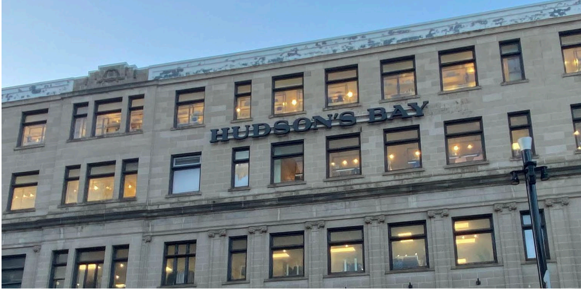
Close up of the upper floors of the five storey section, a decorative medallion the roof level. City of Ottawa, 2024.
