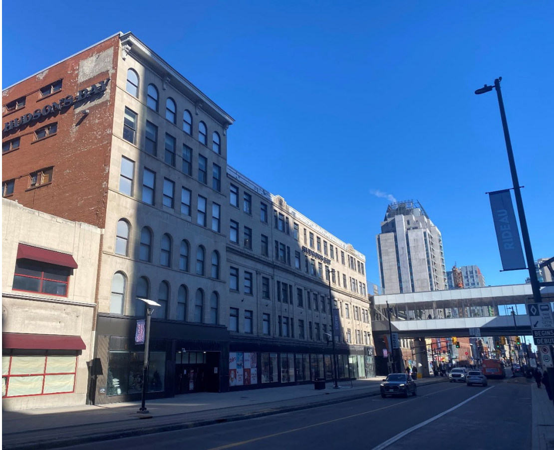
Six-storey portion of 73 Rideau Street, formerly the Stewart Building. City of Ottawa, 2024.
