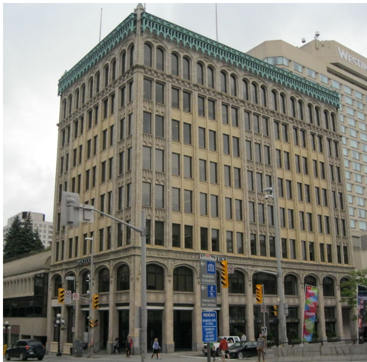
Transportation Building at 10 Rideau Street, City of Ottawa , 2013.
