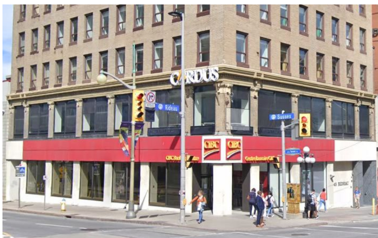
First two storeys of the building showing second storey cornice. Google Maps , 2021.
