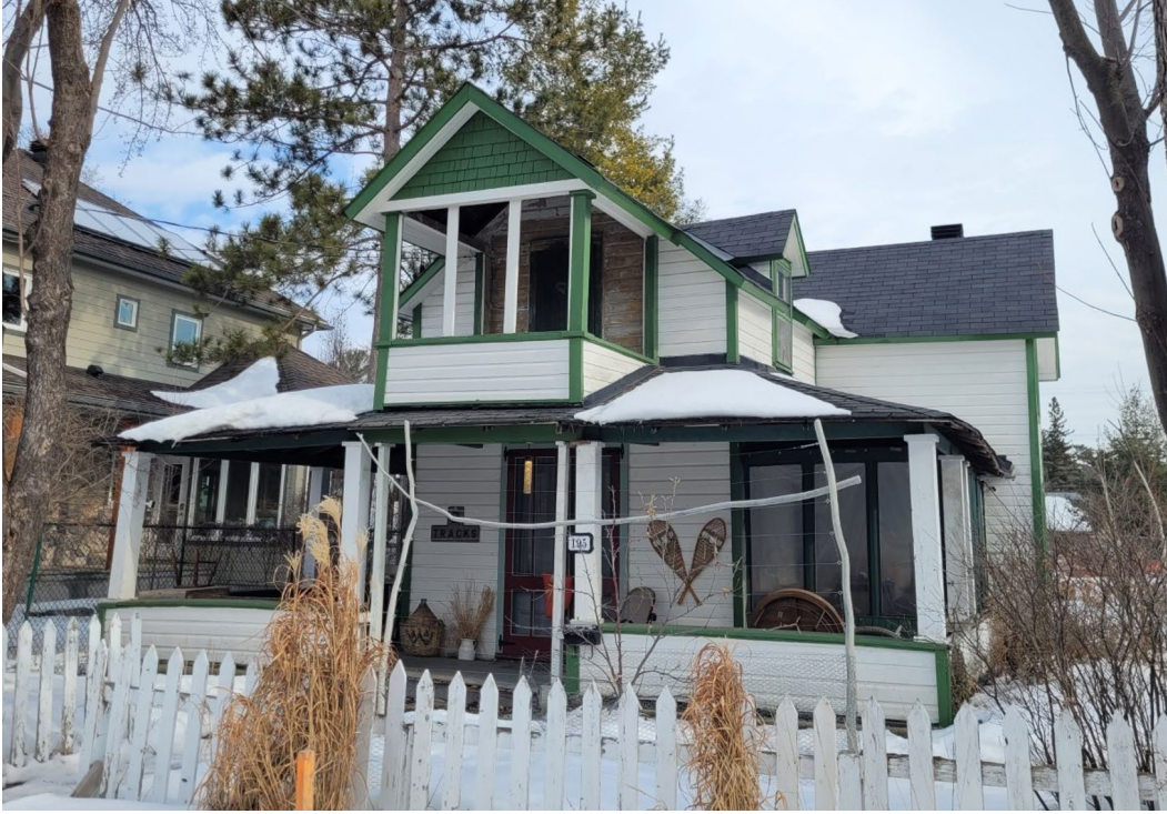
195 Bradford Street. City of Ottawa, 2024
