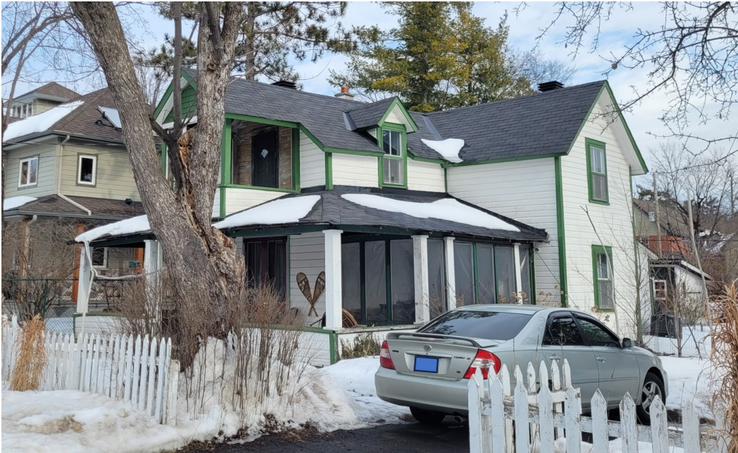
195 Bradford Street. City of Ottawa, 2024
