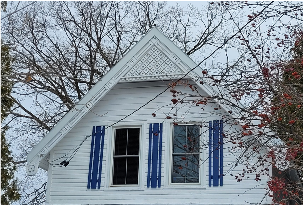
Gable apex panel detail, 119 Bradford Street. City of Ottawa, 2024
