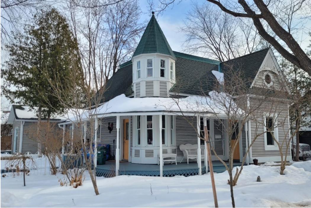
205 Bradford Street. City of Ottawa, 2024
