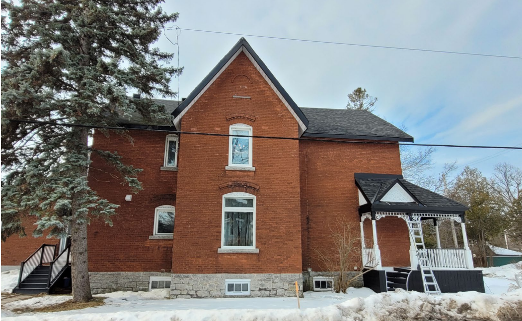
Side façade (east), 2764 Rowatt Street. City of Ottawa, 2024
