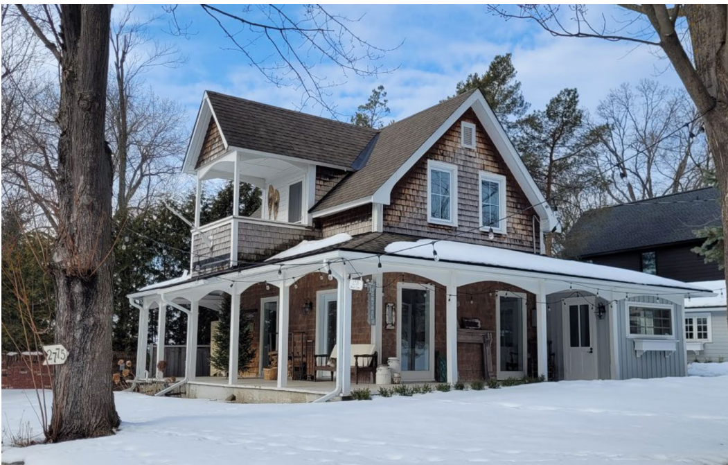
2775 Rowatt Street, City of Ottawa, 2024
