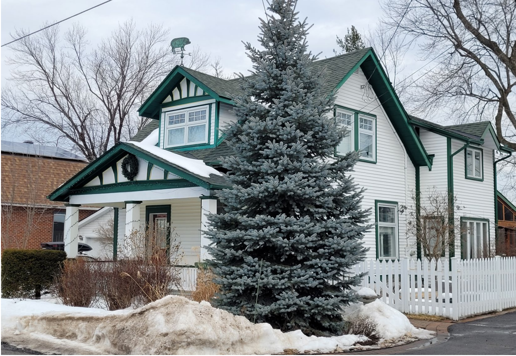
73 Britannia Road. City of Ottawa, 2024
