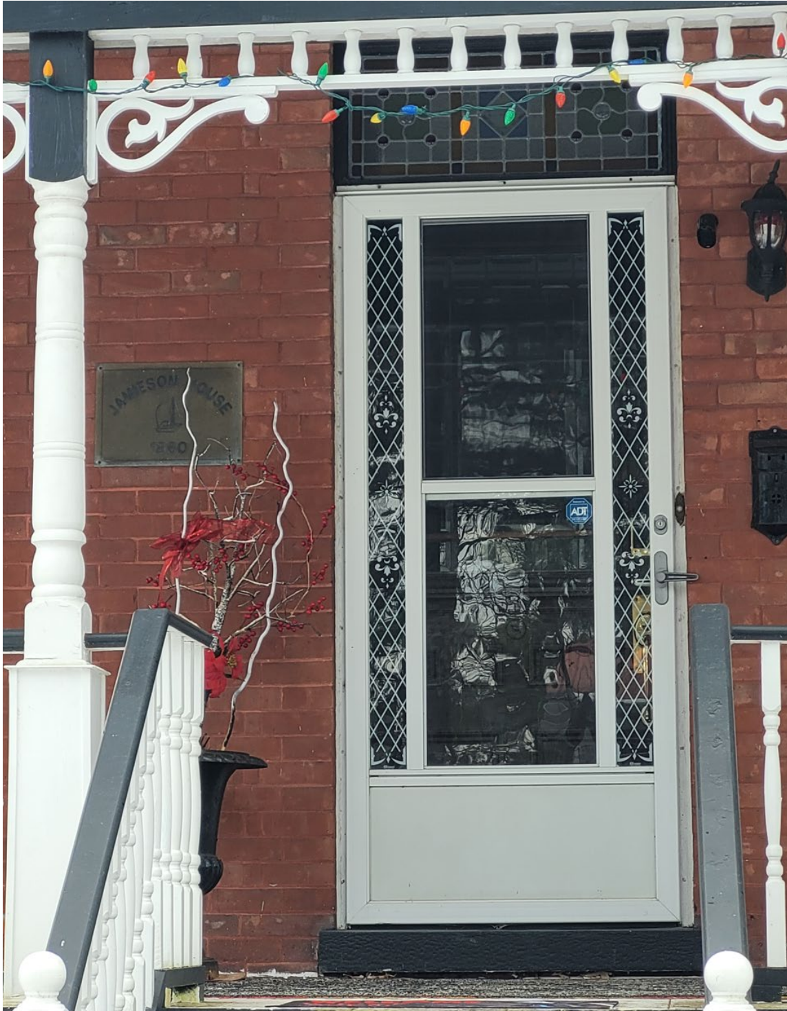
Front entrance detail, 2764 Rowatt Street. City of Ottawa, 2024
