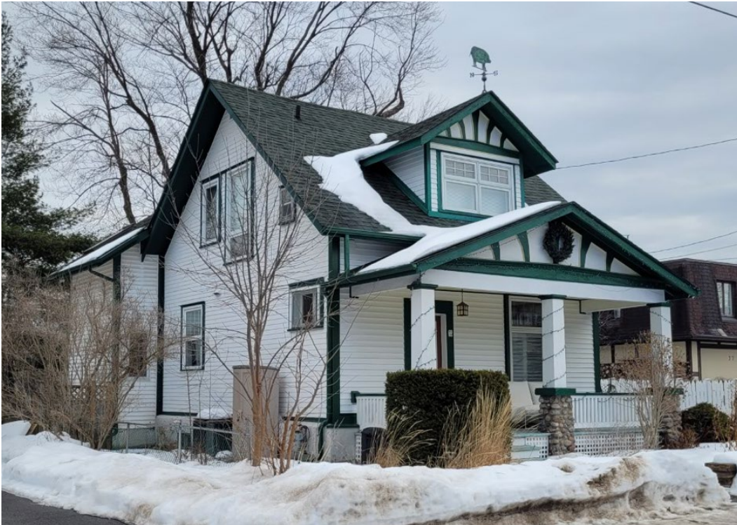
73 Britannia Road. City of Ottawa, 2024
