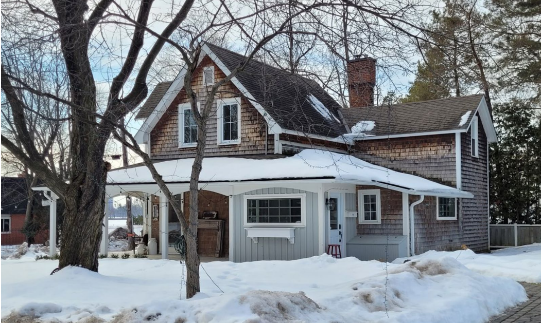
2775 Rowatt Street, City of Ottawa, 2024
