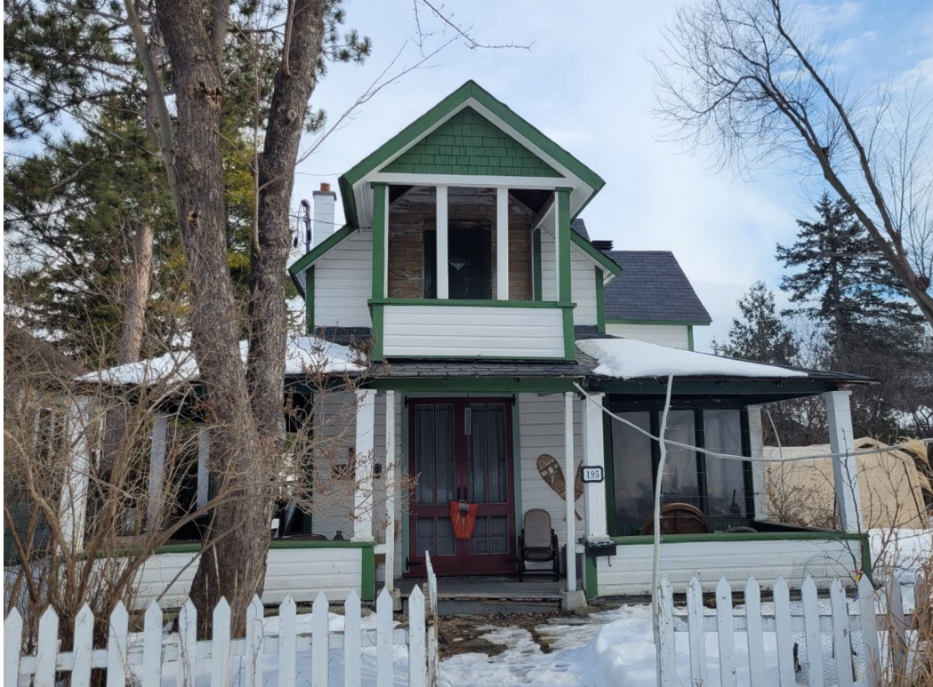
Front façade, 195 Bradford Street. City of Ottawa, 2024
