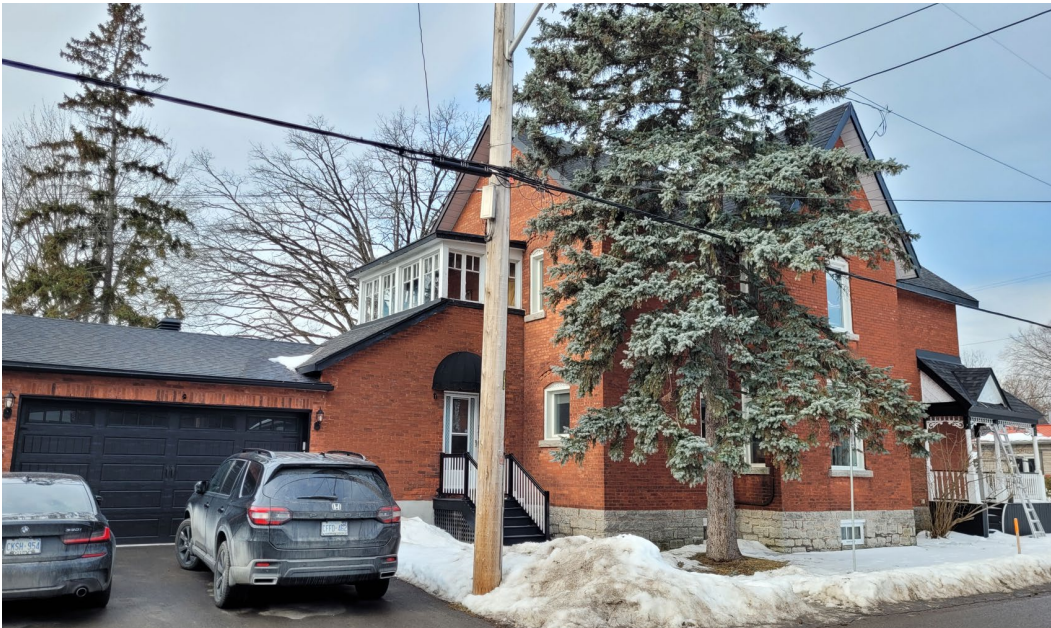
2764 Rowatt Street. City of Ottawa, 2024
