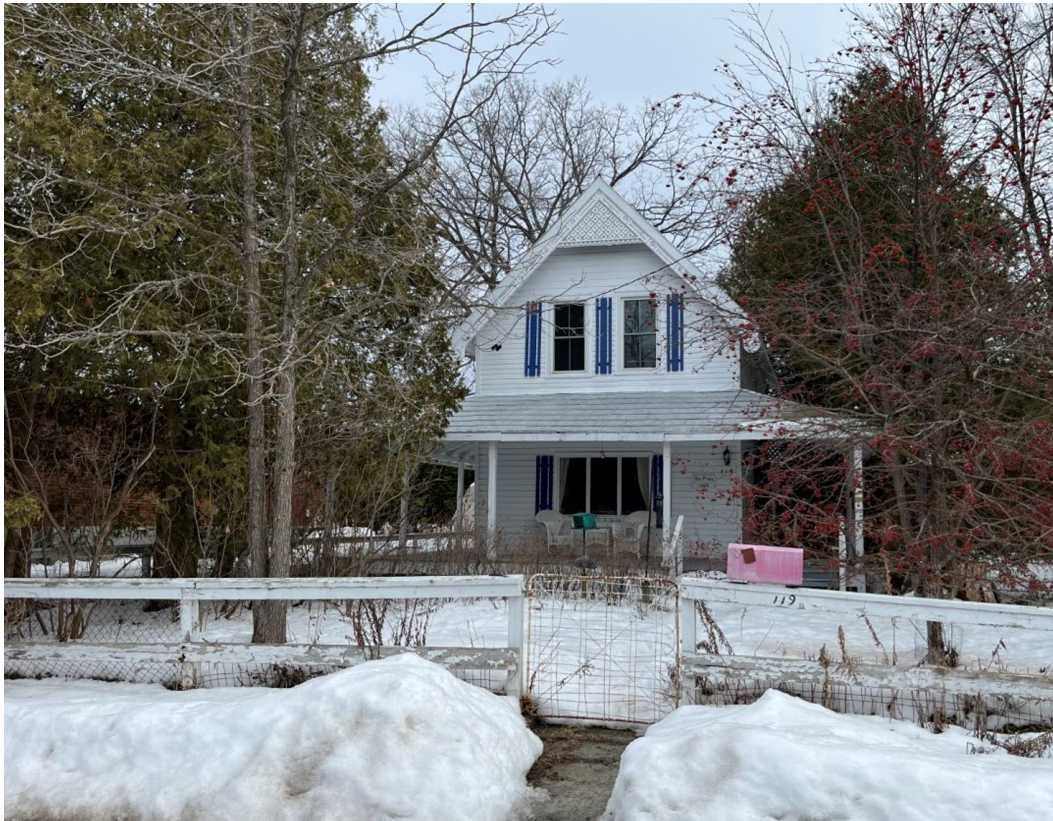
Front façade, 119 Bradford Street. City of Ottawa, 2024
