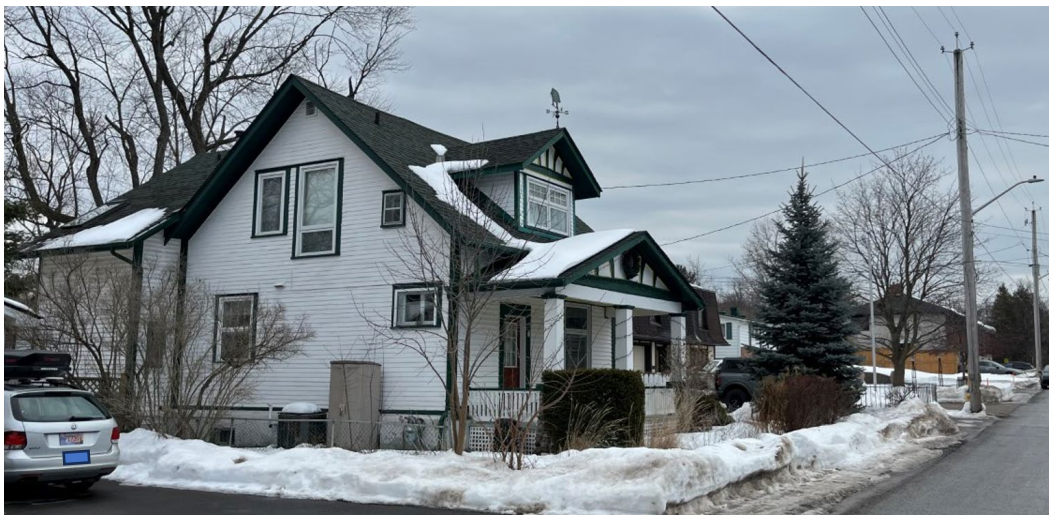
73 Britannia Road. City of Ottawa, 2024
