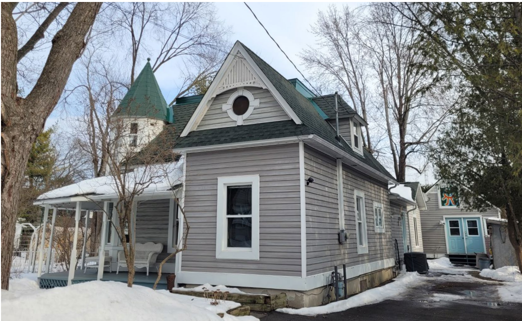
205 Bradford Street. City of Ottawa, 2024
