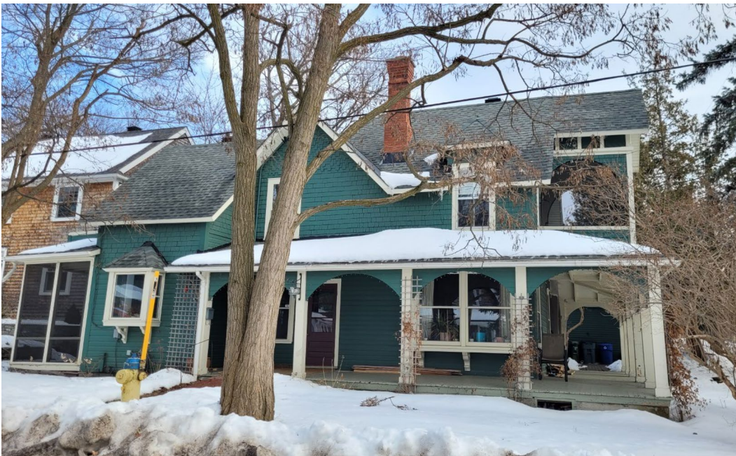
Side elevation (west), 95 Kirby Street. City of Ottawa, 2024
