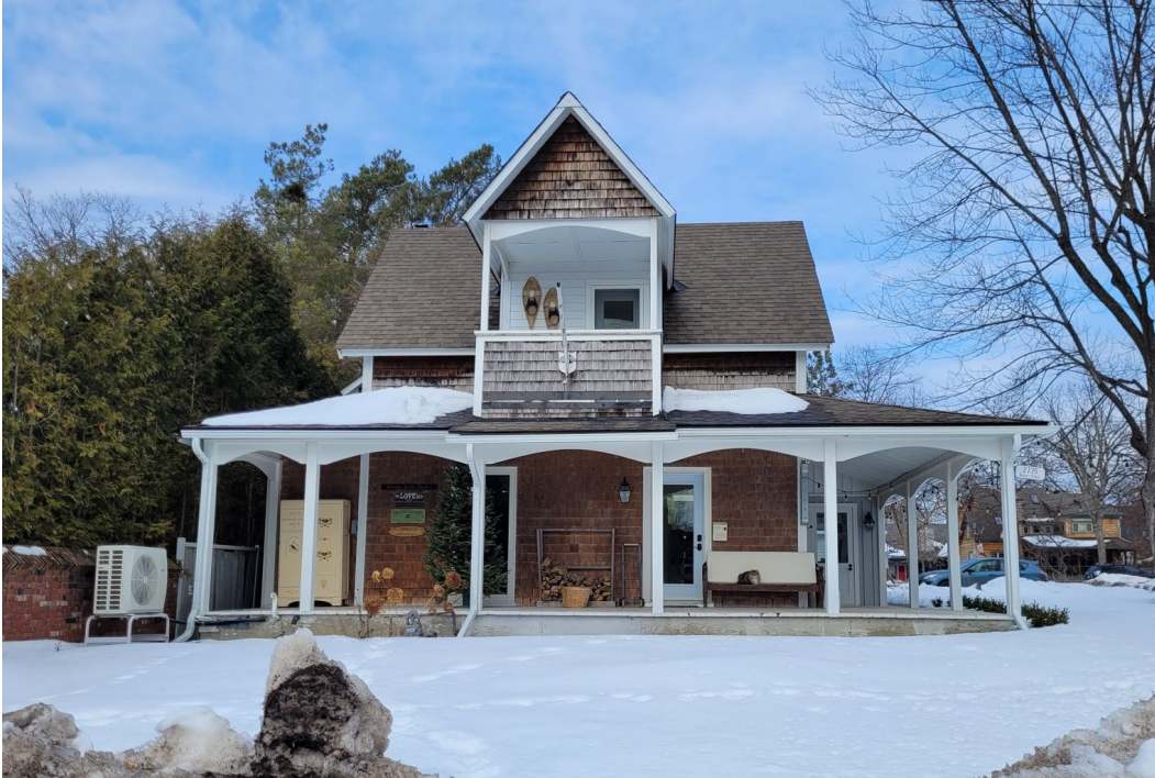
2775 Rowatt Street, City of Ottawa, 2024
