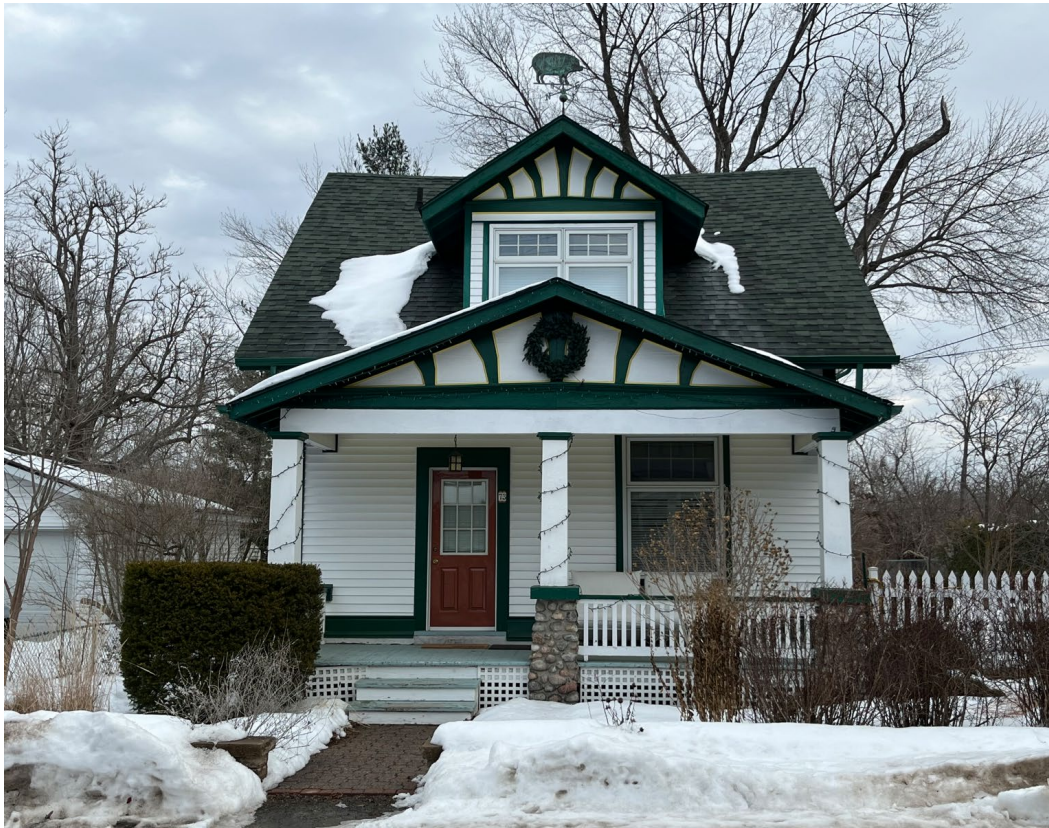
Front façade, 73 Britannia Road. City of Ottawa, 2024
