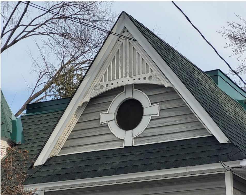
Gable apex panel detail, 205 Bradford Street. City of Ottawa, 2024
