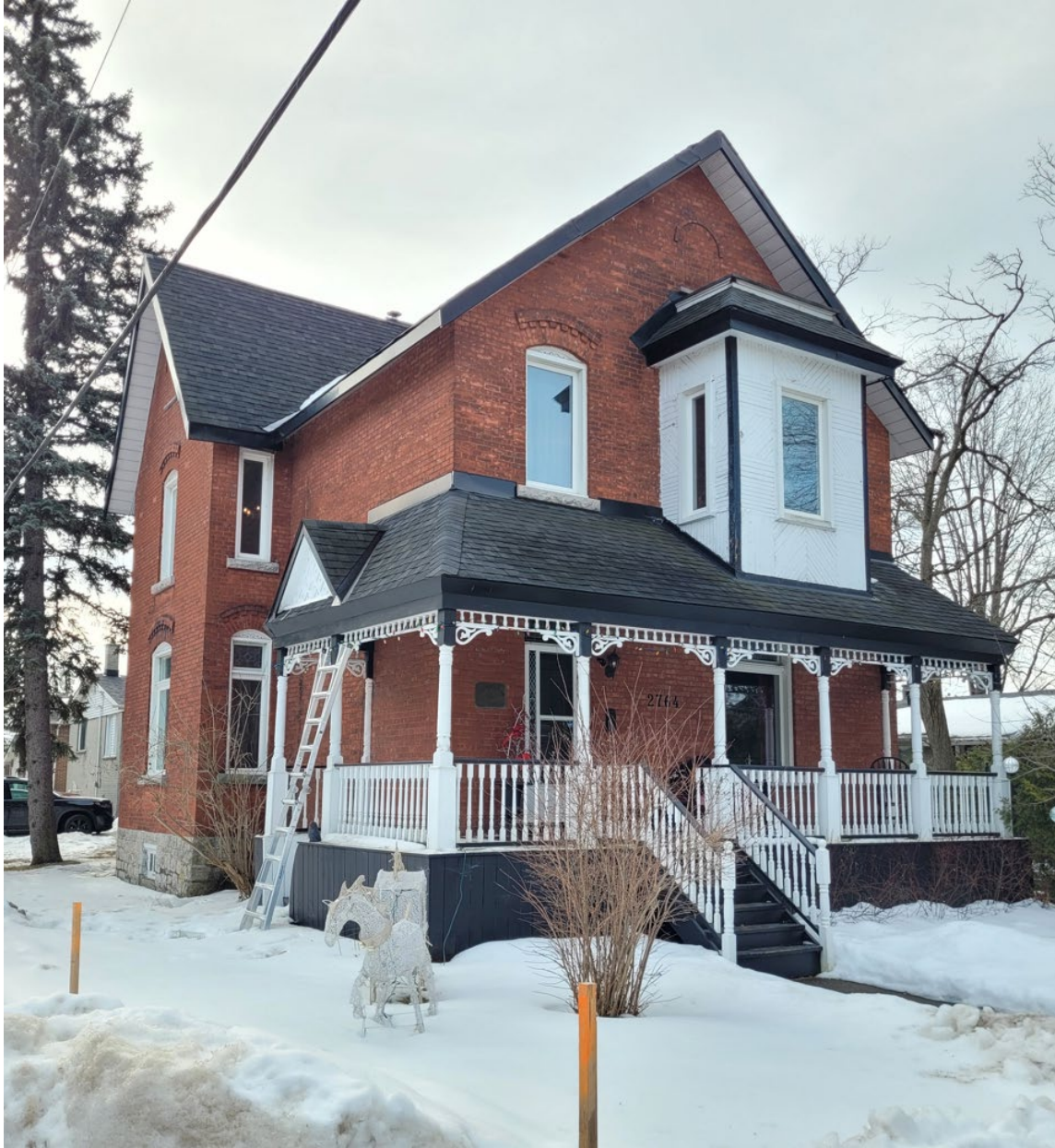
2764 Rowatt Street. City of Ottawa, 2024
