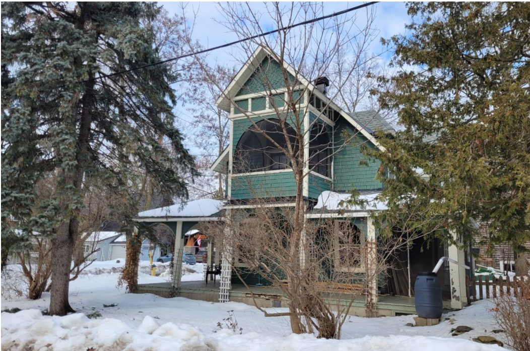
95 Kirby Street. City of Ottawa, 2024
