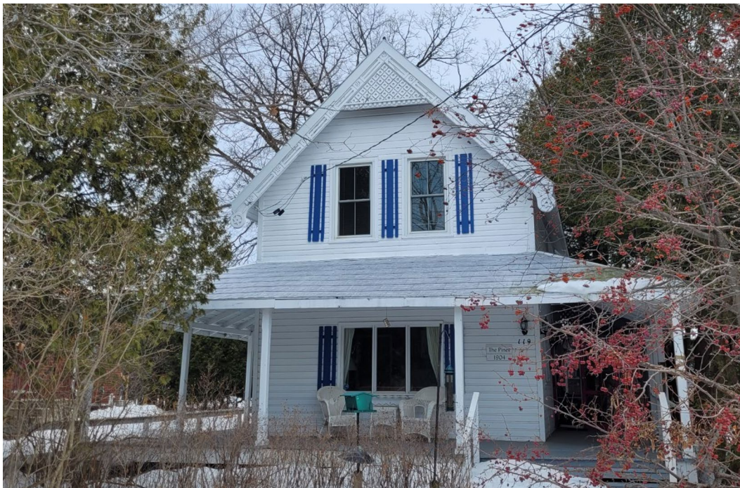
Front façade, 119 Bradford Street. City of Ottawa, 2024
