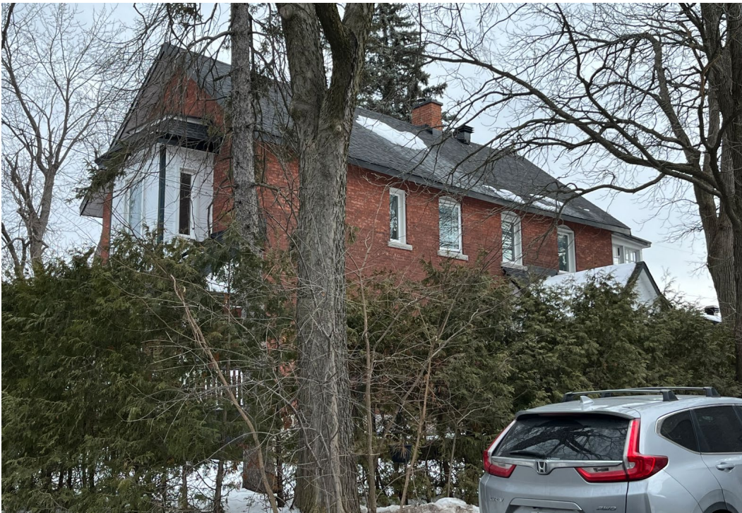
2764 Rowatt Street. City of Ottawa, 2024
