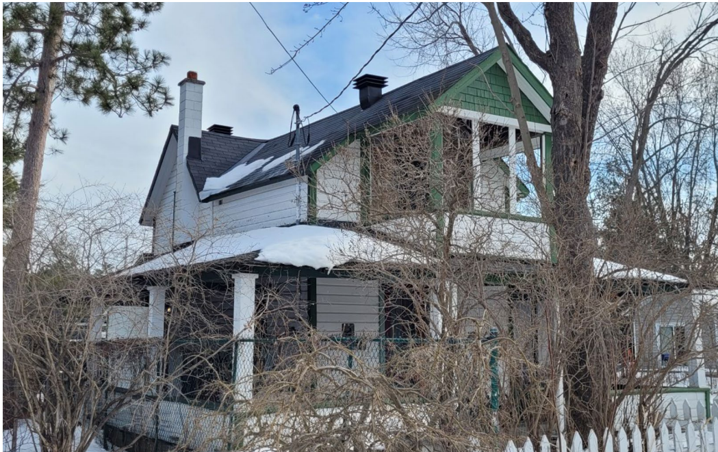
195 Bradford Street. City of Ottawa, 2024
