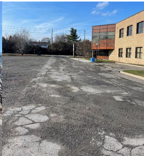
Photo of existing driveway
