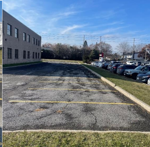
Photo of parking on north side
