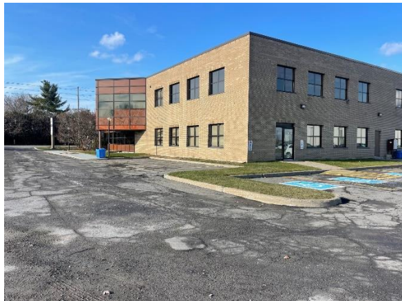
Photo of parking on the south side of Greenbelt Church
