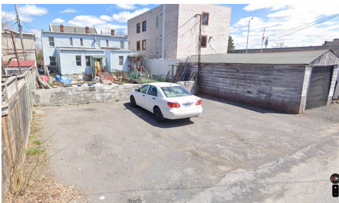
Existing Parking Area
